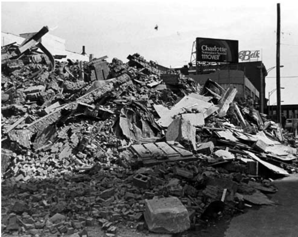
The Independence Building was reduced to rubble in September 1981.
