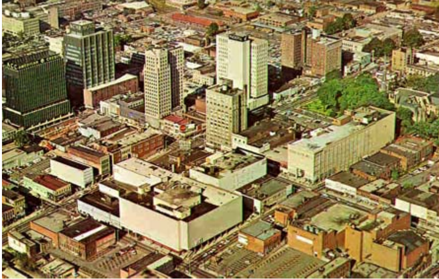
This 1966 photograph shows the North Carolina National Bank Building and the Cutter Building before they were altered. The Wachovia Bank and Trust Company Building looms over W. Trade St. The arcade portion of the Builders Building is clearly visible.
