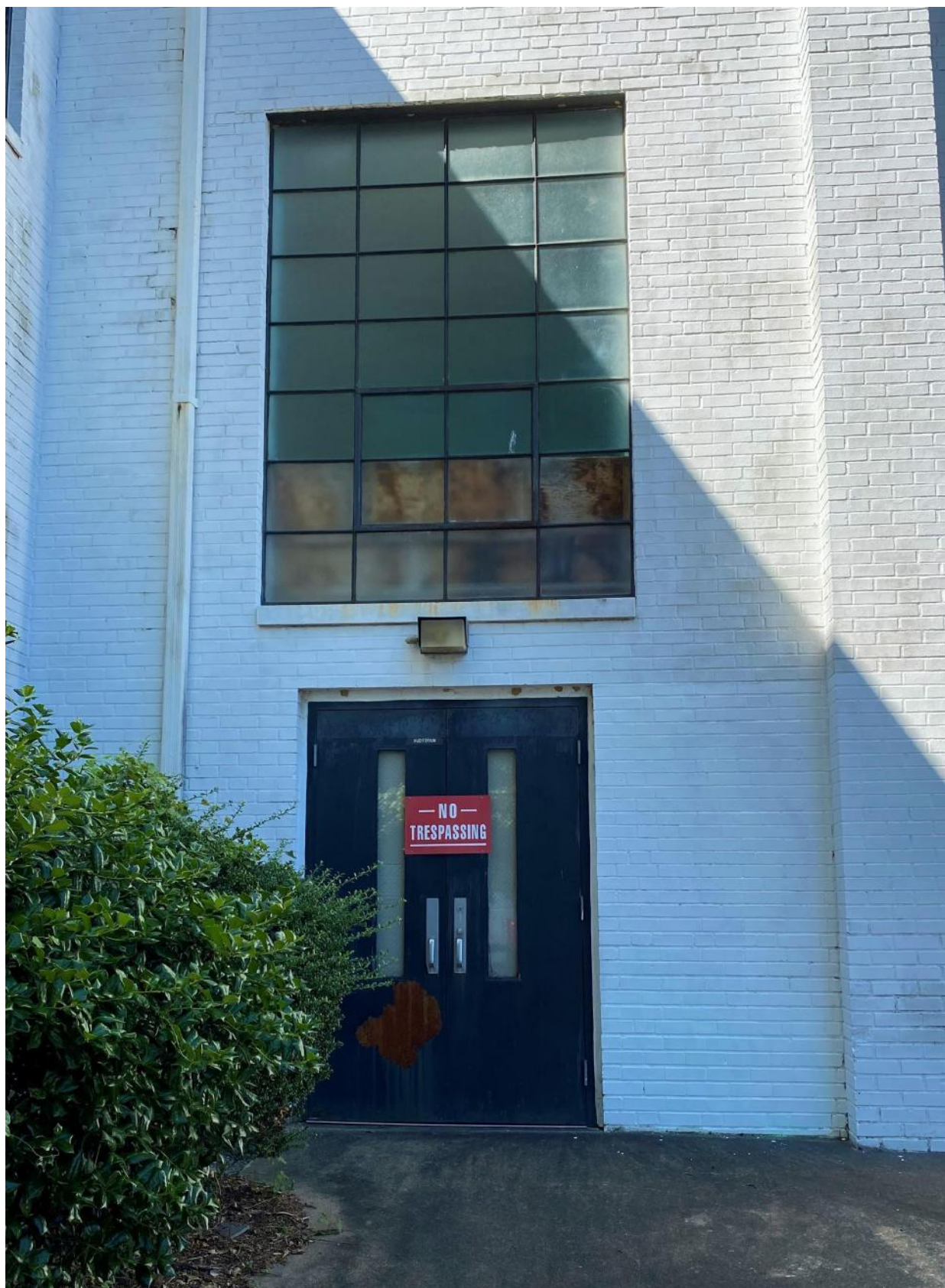
Fig. 12f: Side (East) Elevation Door
