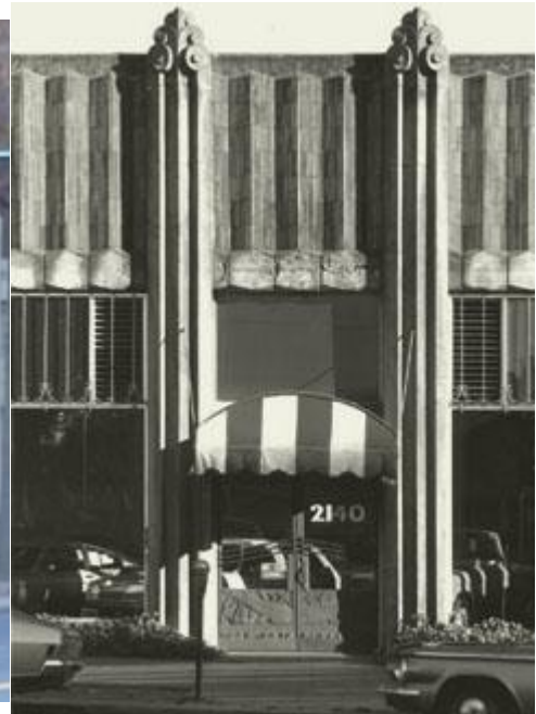
Art Deco landmark Howard Automobile Co. Showroom, 1930, Berkeley, CA
