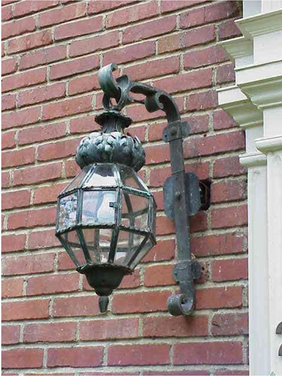
Original light fixtures
