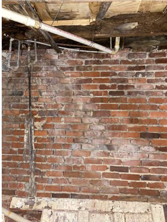
Rear Foundation Deterioration
