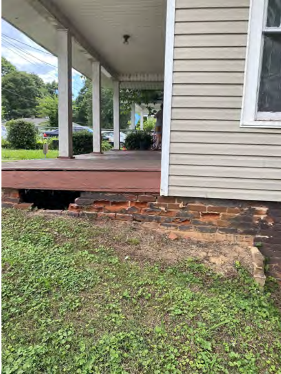
Side Foundation Deterioration
