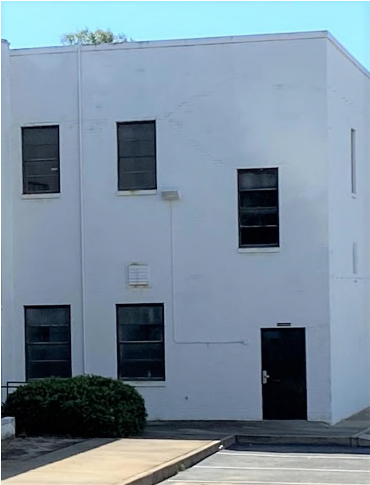
Fig. 11c: Two-over-two metal framed windows
