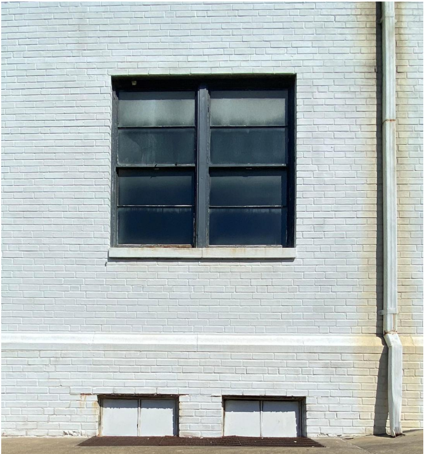
Fig. 11b: Two-over-two metal framed windows
