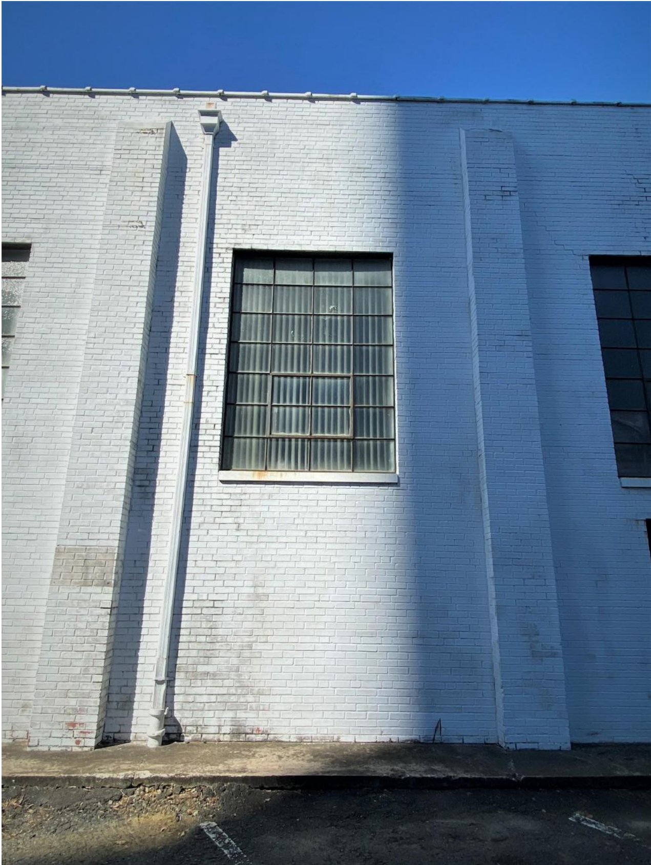
Fig. 10: Exterior Brick Columns
