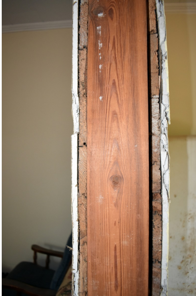
Figure 13 The cased opening between the left two bedrooms has been temporarily removed. Visible are the original ca. 1902 tongue-and-groove wood board walls (right) and the ca. 1920s tongue-and-groove board covered walls (right) covered with ca. 1950s gypsum wall board.
