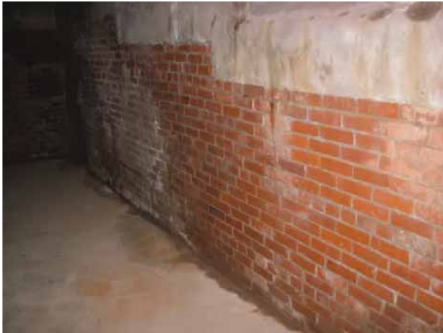
Photo #17: Addition of basement level under original stepped concrete footing.
