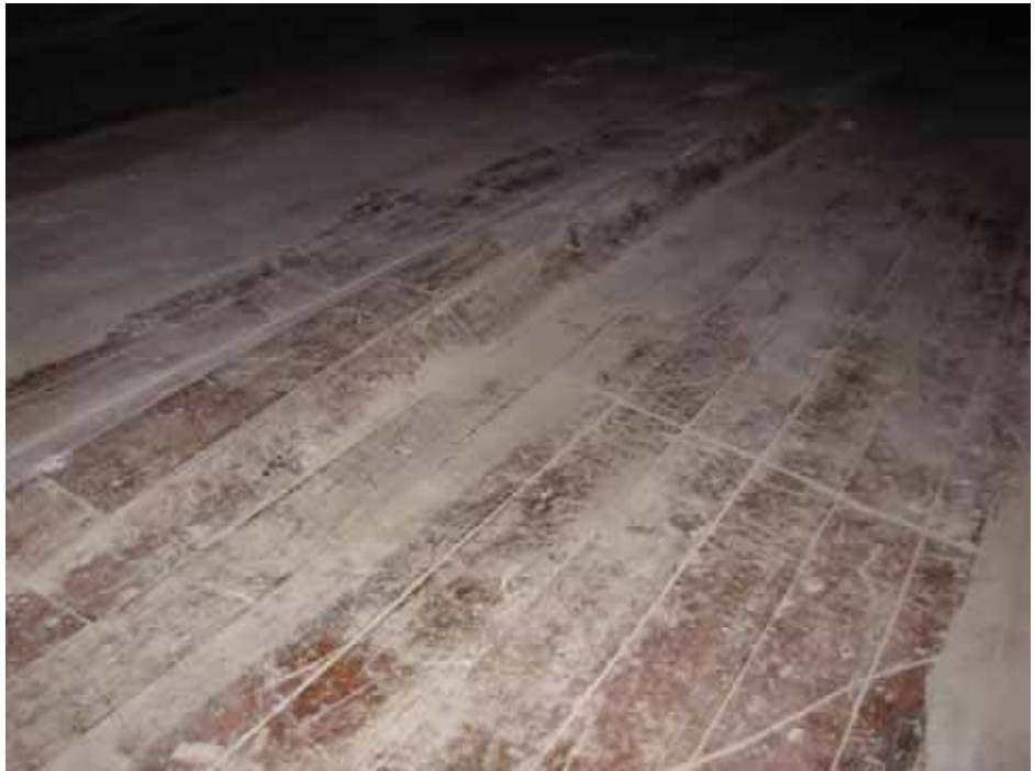
Photo #13: Buckled finished pine flooring likely due to water damage that could have deteriorated structural wood decking below.
