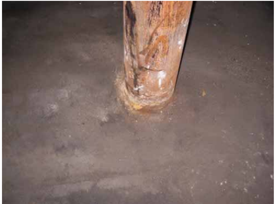
Photo #19: Compacted coal fines and no evident sign of footing size or existence.
