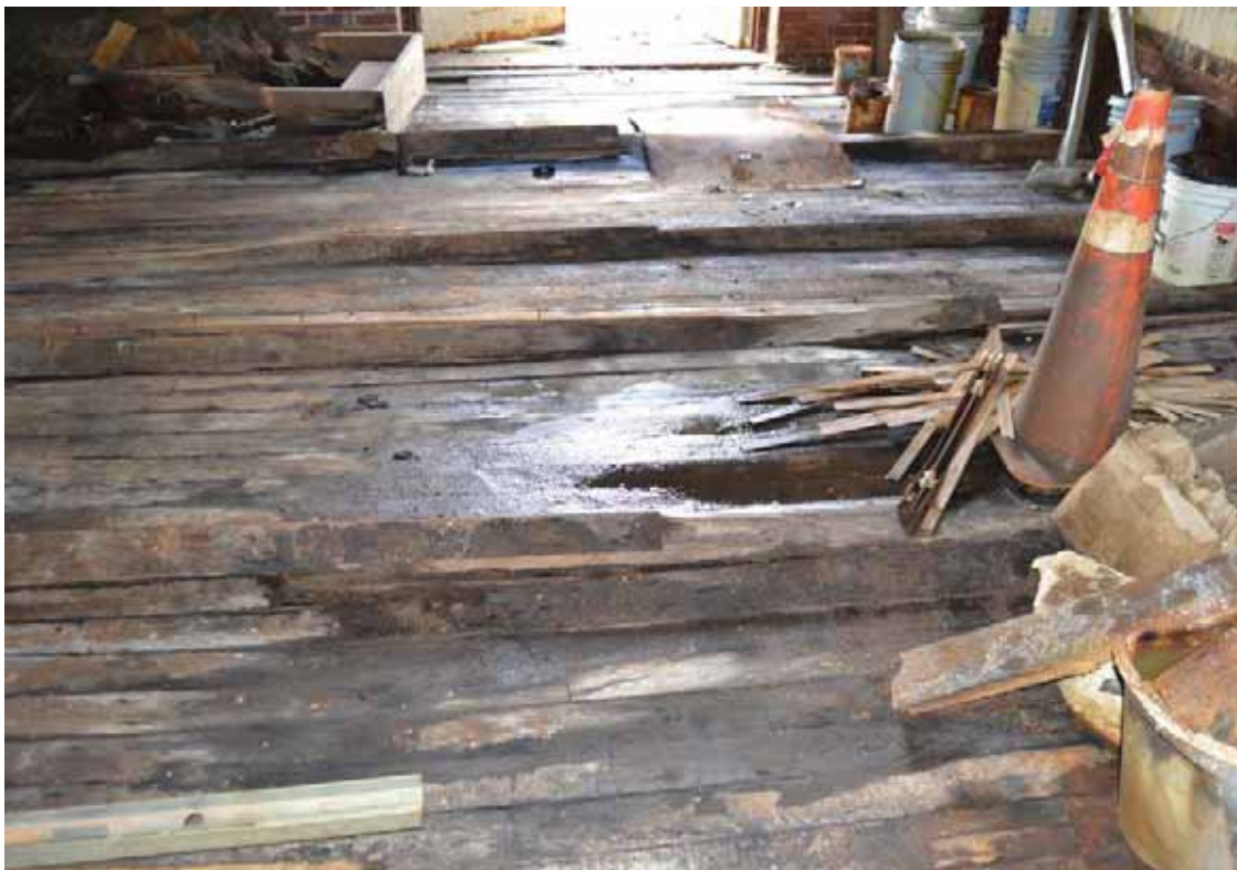
40. First floor, damaged floor structure in south wing
