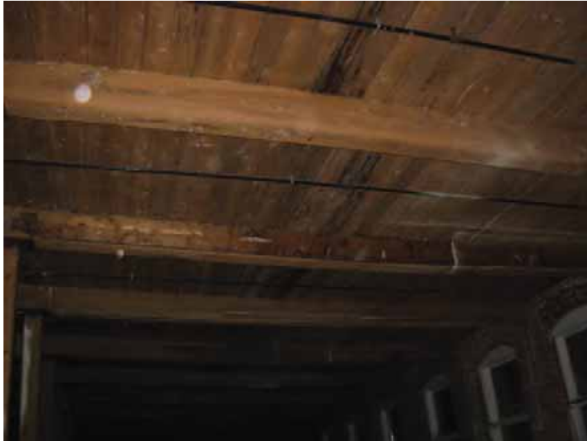
Photo #7: Dimensional lumber used to reinforce existing timber beam. Reinforcing likely used to stabilize member due to damages.
