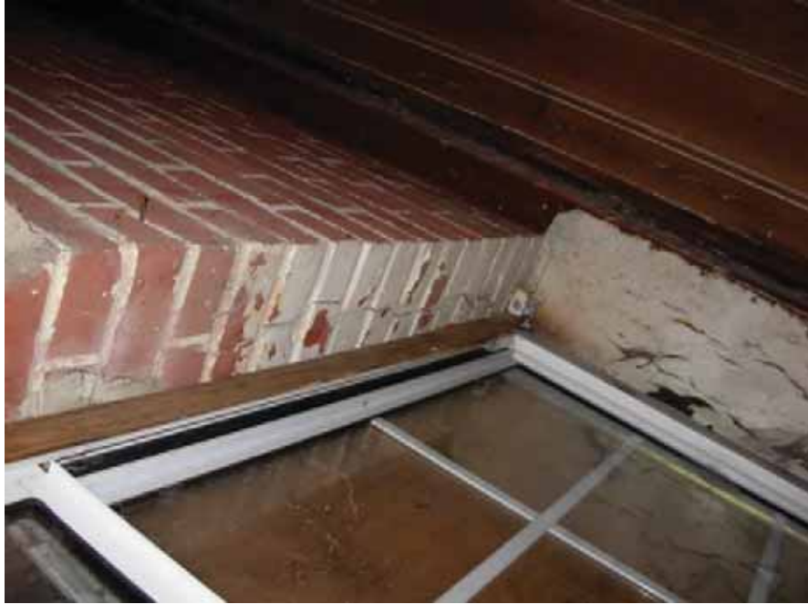
Photo #15: Cracking in brick that needs repair.
