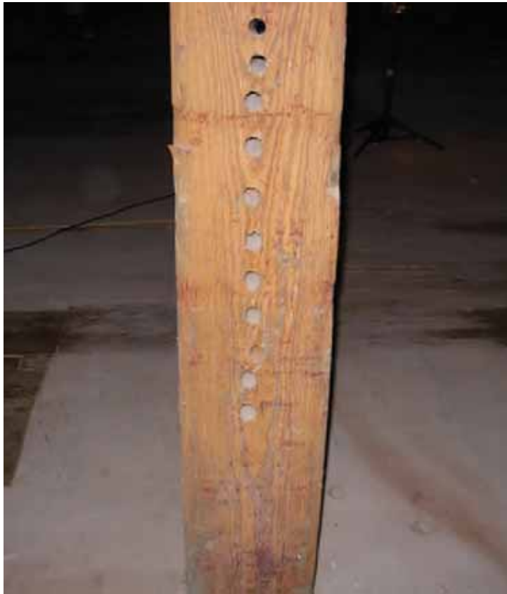
Photo #3: Excessive reduction in column cross section due to improper modification during utility routing.
