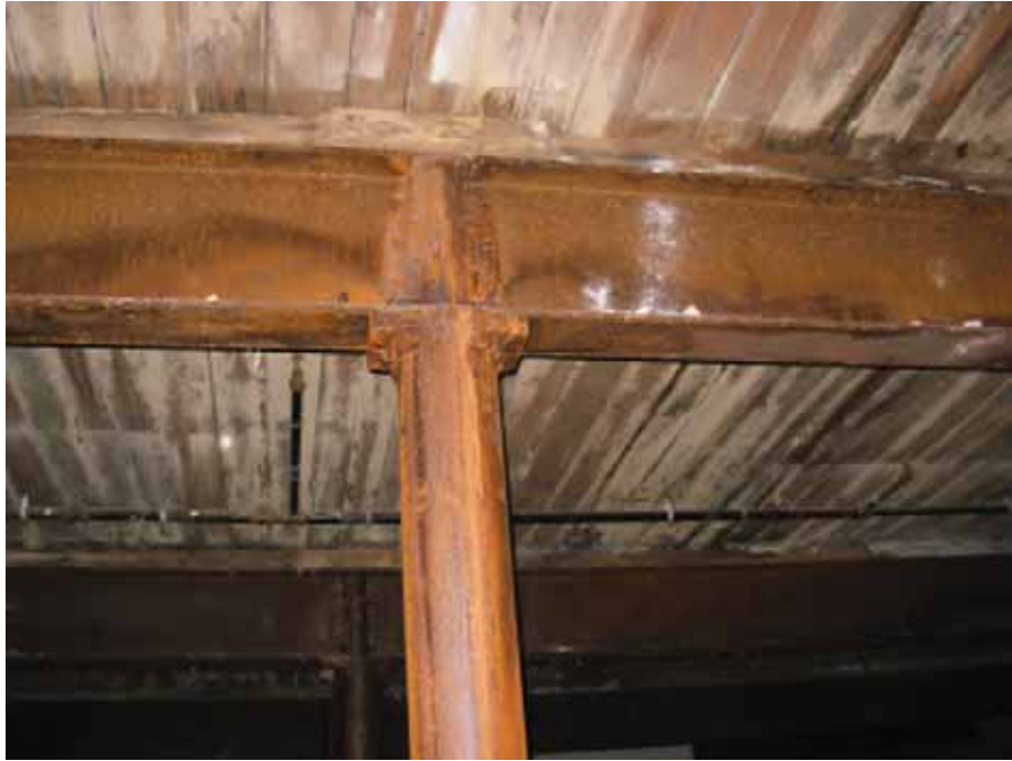
Photo #1: Typical steel framing at column and beam connections.
