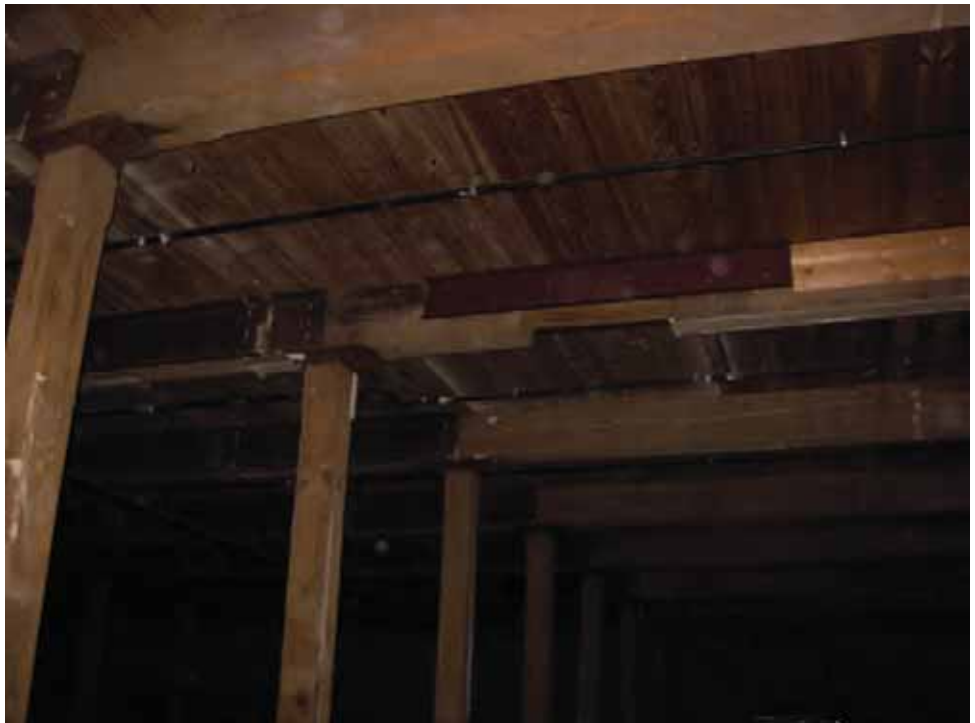
Photo #8: Small partial length steel channel and dimensional lumber reinforcing around large notch in wooden beam.
