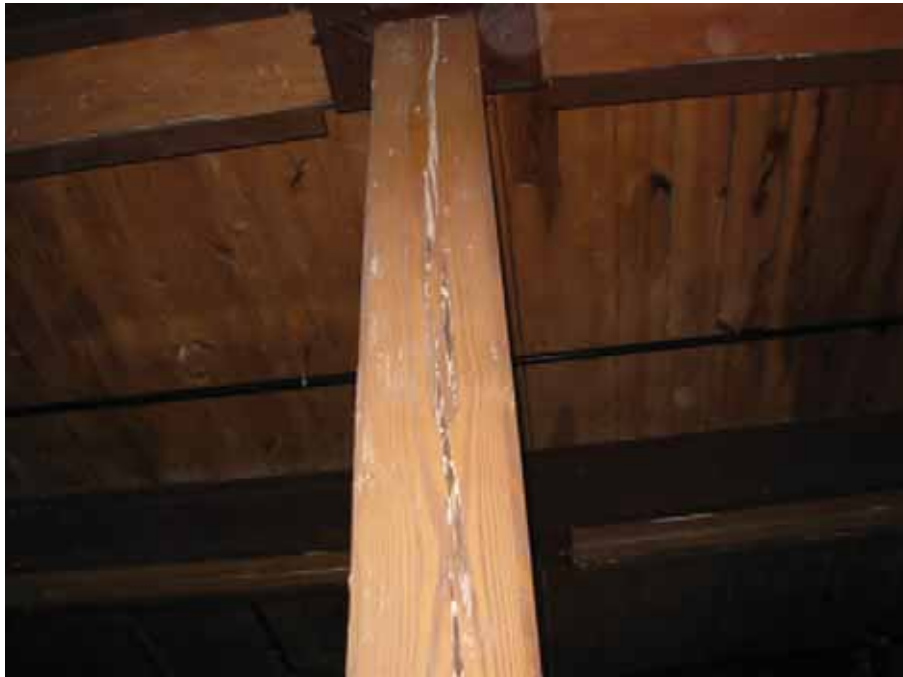
Photo #5: Large checks in wooden column. White filler material assumed to be drywall joint compound and not an attempt to epoxy the cracks.
