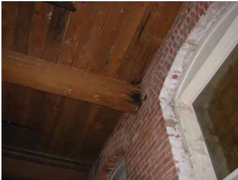
Photo #10: Rotten end of timber at masonry bearing condition.
