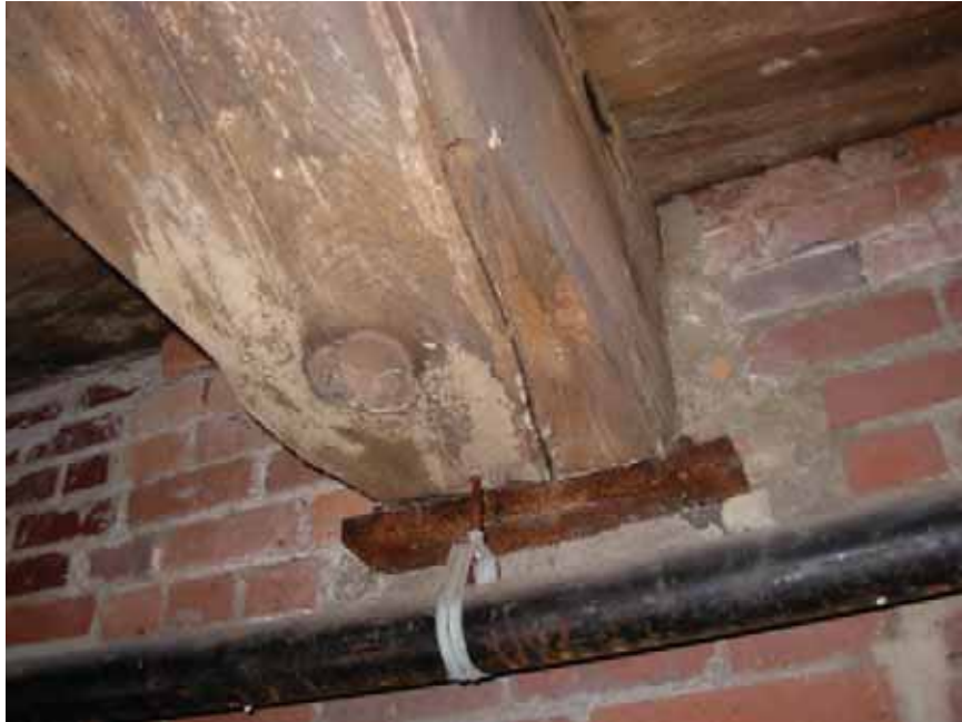
Photo #11: Severe checking in beam. This particular check spirals about the length of the beam and the member needs to be replaced.
