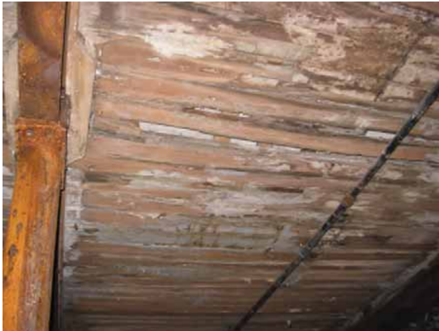
Photo #12: Steel structure shows heavy surface rusting but appears to be sound although wood decking needs to be removed and replaced.
