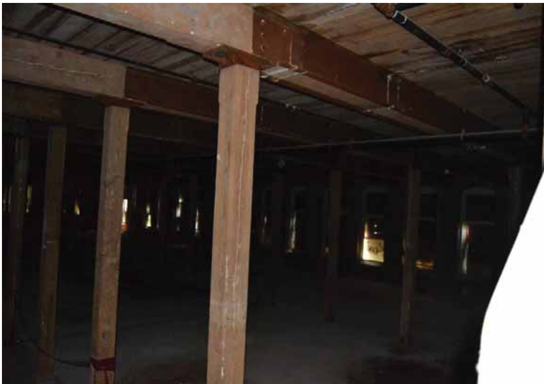
55. First floor, south wing, detail of steel reinforced timbers
