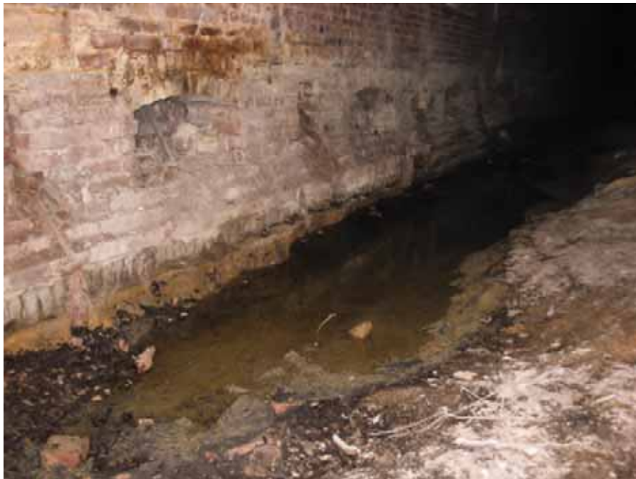
Photo #18: Removed wooden framing at crawlspace area and exposed continuous exterior wall footing which has been undermined by water intrusion.
