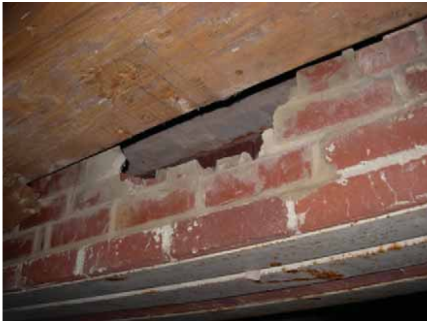
Photo #14: Opening in brick likely for utility routing that needs to be repaired.
