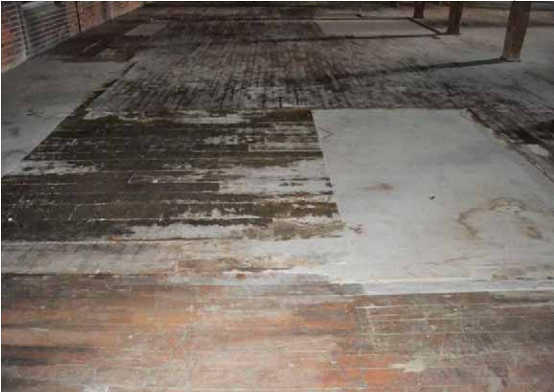
66. Second floor, original portion, detail of flooring structure and infills
