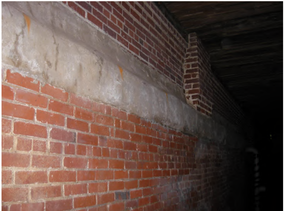
Photo #16: Addition of basement level below continuous footing.
