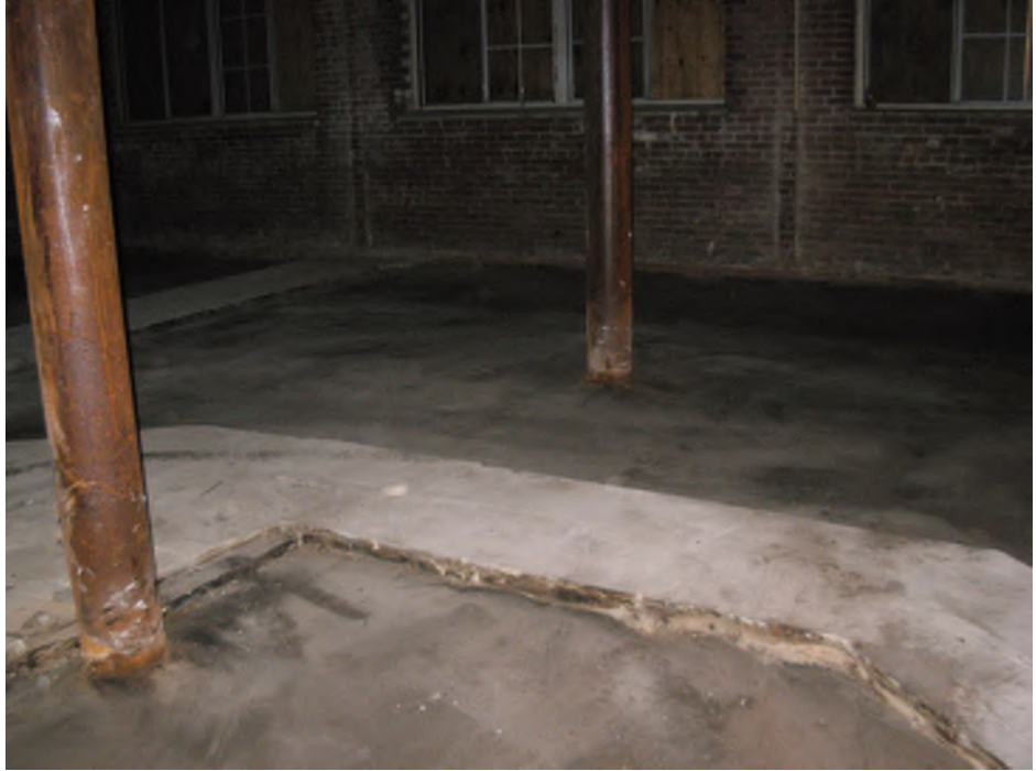
Photo #21: Continuous footings possibly from previous renovation to support load bearing walls.
