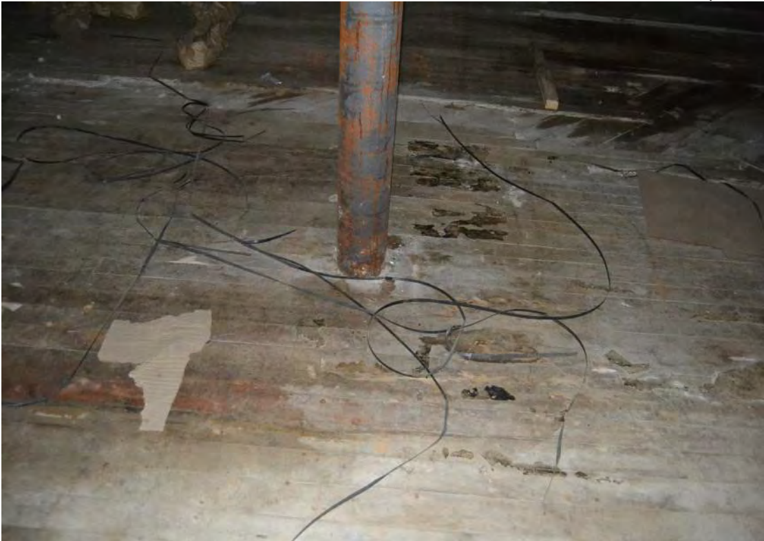
43. First floor, south wing, steel column and floor structure detail; evidence for former gypsum concrete at right
