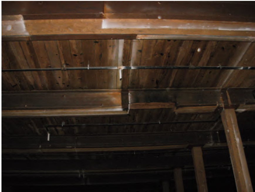
Photo #9: Typical full length channel reinforcing on each side of timber beams. Note the unacceptable torch cut notch in the bottom of the beam. This is a critical section of the beam and should not be notched to this extent.
