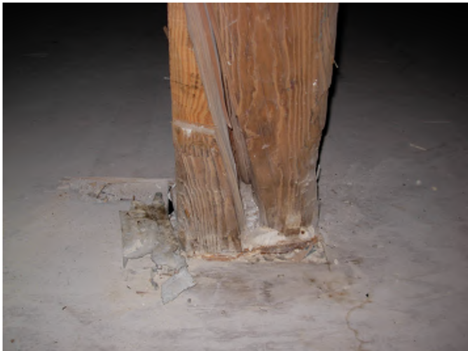
Photo #6: Damaged column base either from impact or overloading. Column needs replacement.
