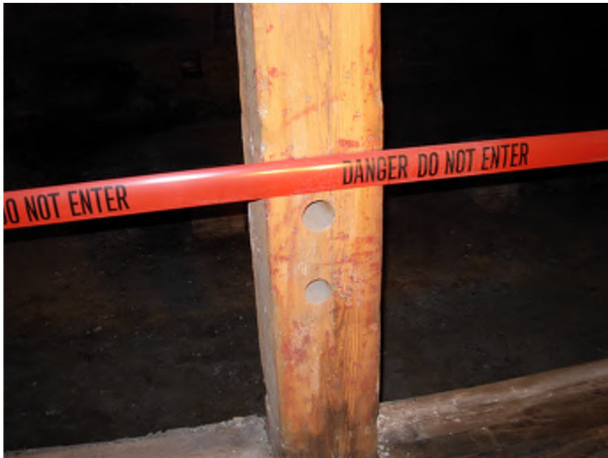
Photo #4: Multiple large 2" diameter holes in column for utility routing. Excessive reduction in member cross sectional area is unacceptable.
