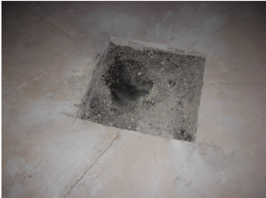
Photo #20: Test location of on grade flooring in basement. Notice the numerous large cracks.
