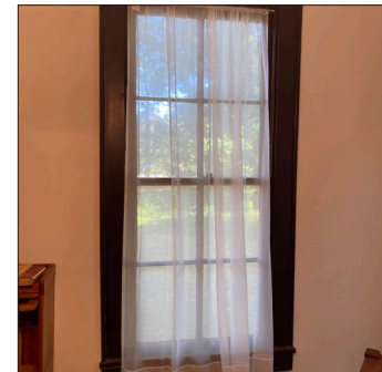
4: REMOVE EXISTING NON-HISTORICAL WINDOW; REPLACE WITH DIVIDED LITE REPLICA TO MATCH ORIGINAL HOUSE
