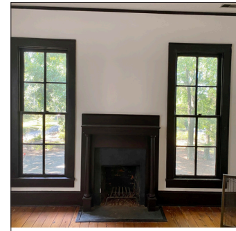
4: REMOVE EXISTING NON-HIS- TORICAL WINDOW; REPLACE WITH DIVIDED LITE REPLICA TO MATCH ORIGINAL HOUSE
