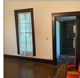
8: REMOVE EXISTING NON-HISTORICAL WINDOW; REPLACE WITH DIVIDED LITE REPLICA TO MATCH ORIGINAL HOUSE
