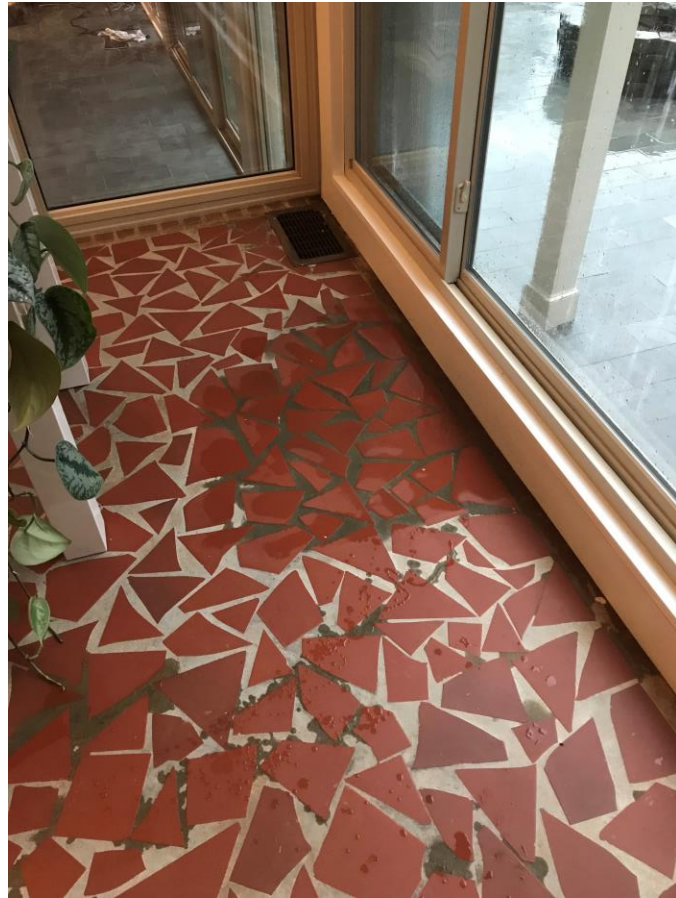
Water penetration through office windows in rear of home
