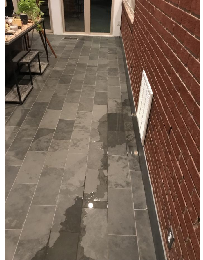
Water pooling in lower level
