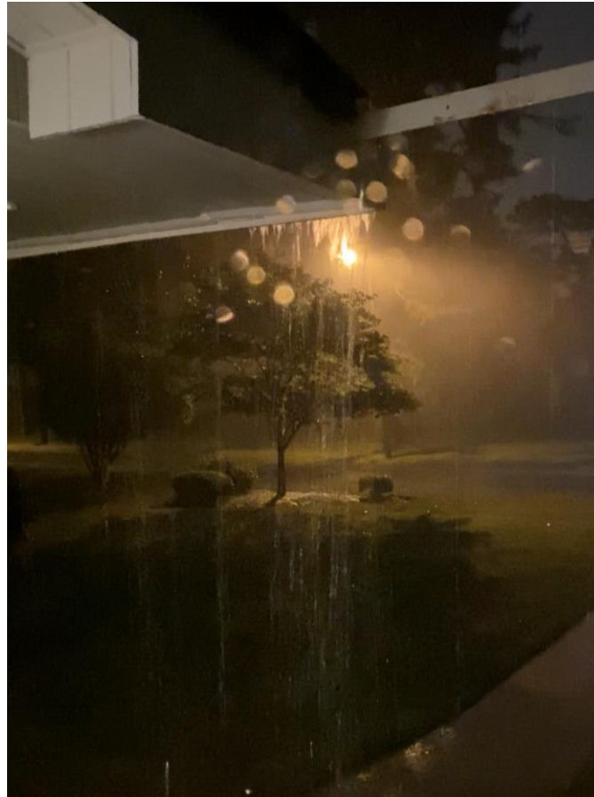
Improperly sloped gutters resulting in overflowing, erosion and wood rot
