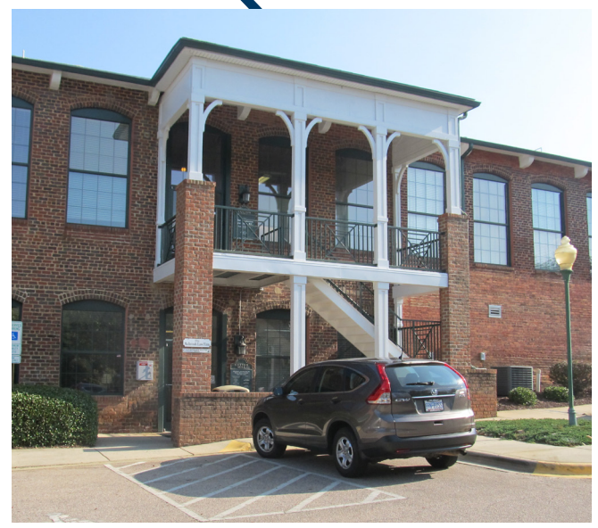
DEMOLISH EXISTING STAIRWAY - 1990'S ADDITION
