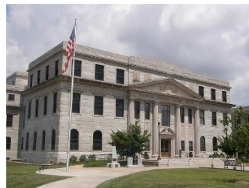
Haywood County Court House.
