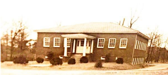
Derita High School Agriculture Building
