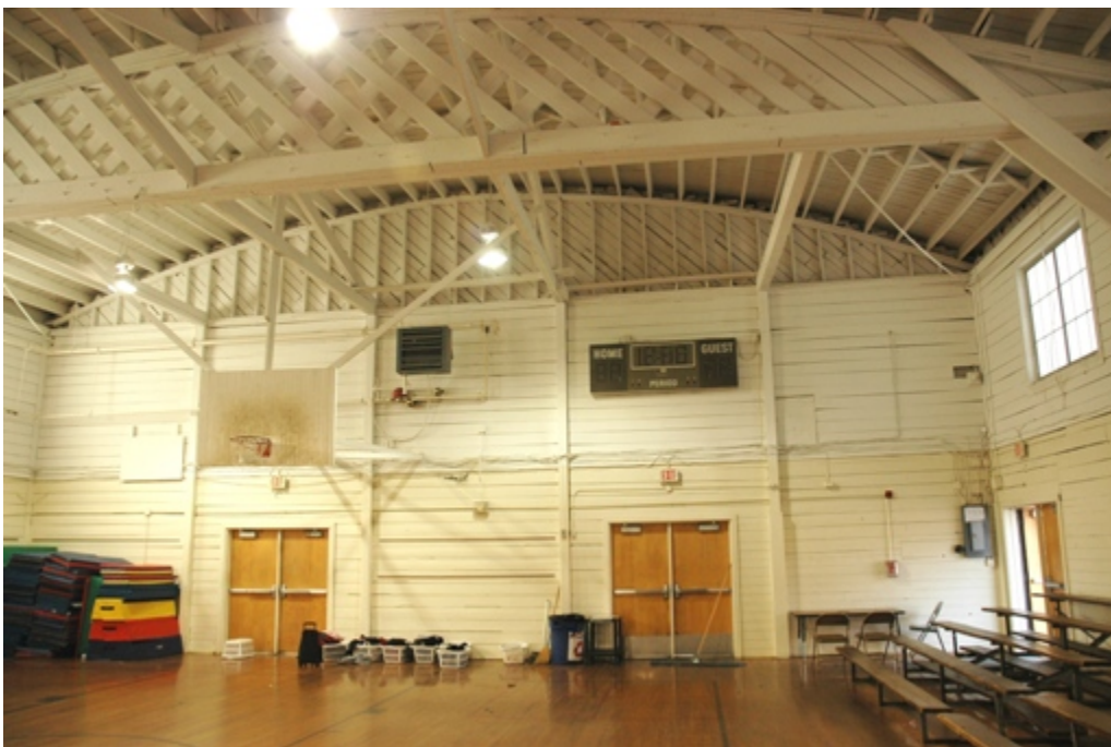
Interior of the 1934 Long Creek Gymnasium
