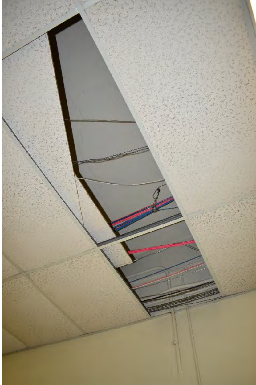
Plaster ceiling visible under acoustic tile ceiling in the first floor hallway of the original 1925 building.
