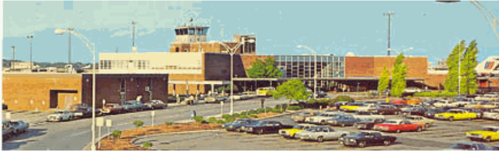
New Terminal designed by Walter Hook, dedicated 1954
