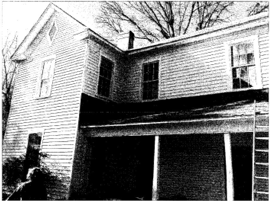
Front/South façade. Wing on left and log portion on right.
