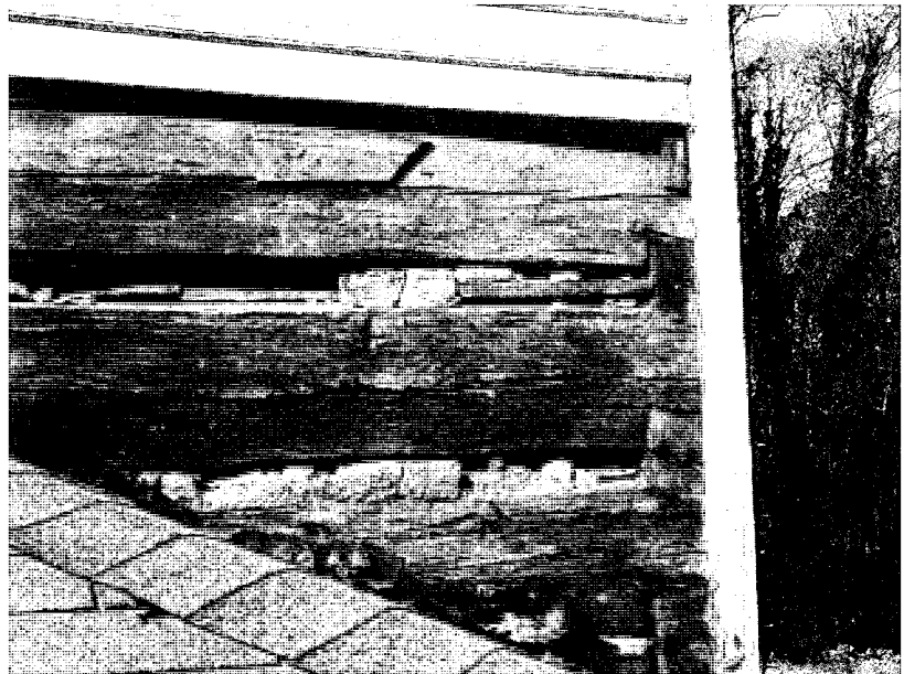
Front/southeast corner of second story(hip of porch roof running across lower left corner), three courses of logs with chinking and half-dovetail notching under clapboards.
