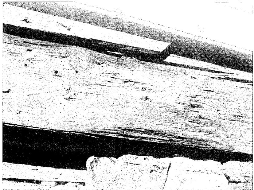
South façade of log portion, just above porch roof. Detail of draw knife marks on log and chinking.
