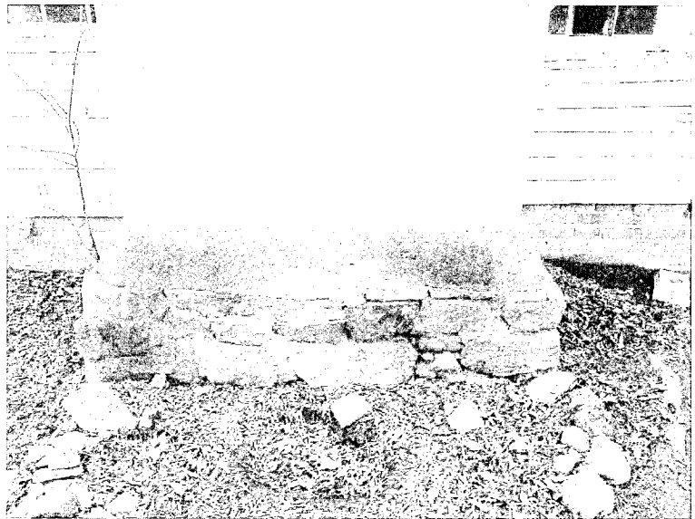
Fieldstone base of east gable end chimney.
