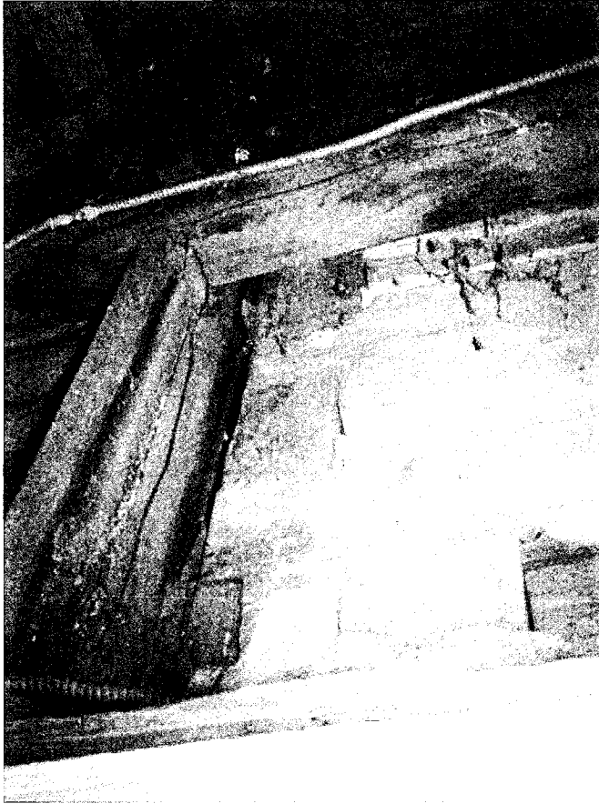
The rear wall (northeast corner) of the log house, viewed from the attic of the Ell, showing courses of logs, half-dovetail notching and whitewash.
