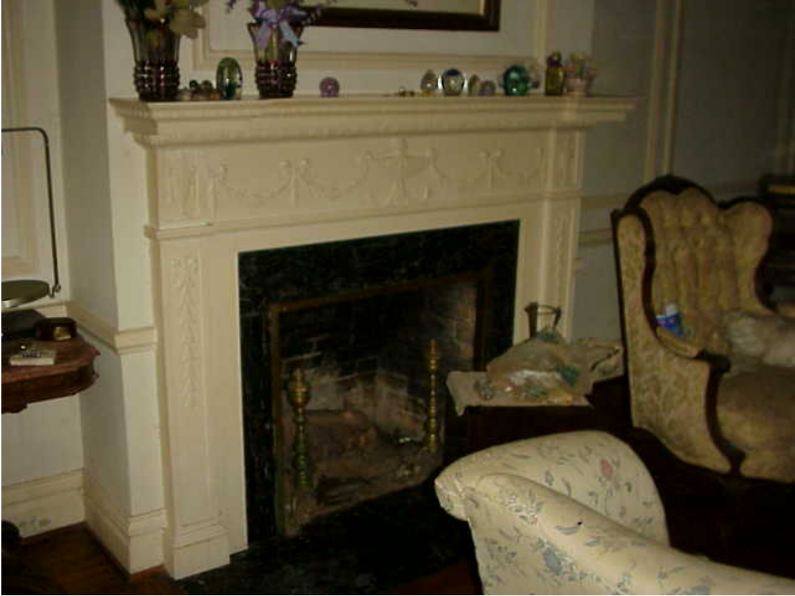
Original woodwork has been preserved
