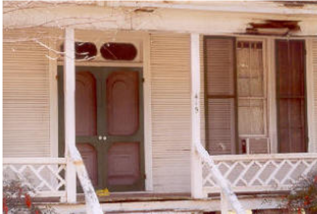
Detail of Front Porch
