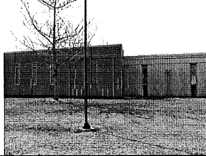
Details of sections added to the façade.
