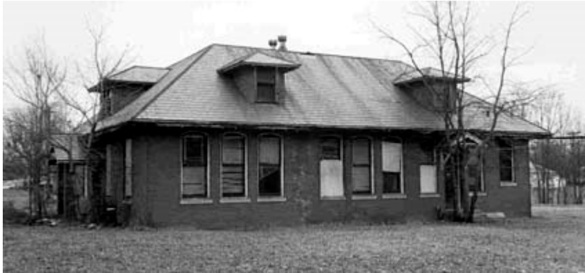
The office building at the Hoskins Mill
