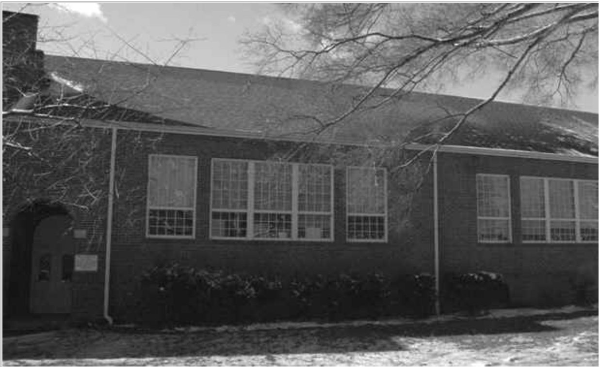
To the south, the next six bays can be divided into two identical sets of three bays. The center bay in each set contains three windows ganged together. The center window is a twenty-five-
