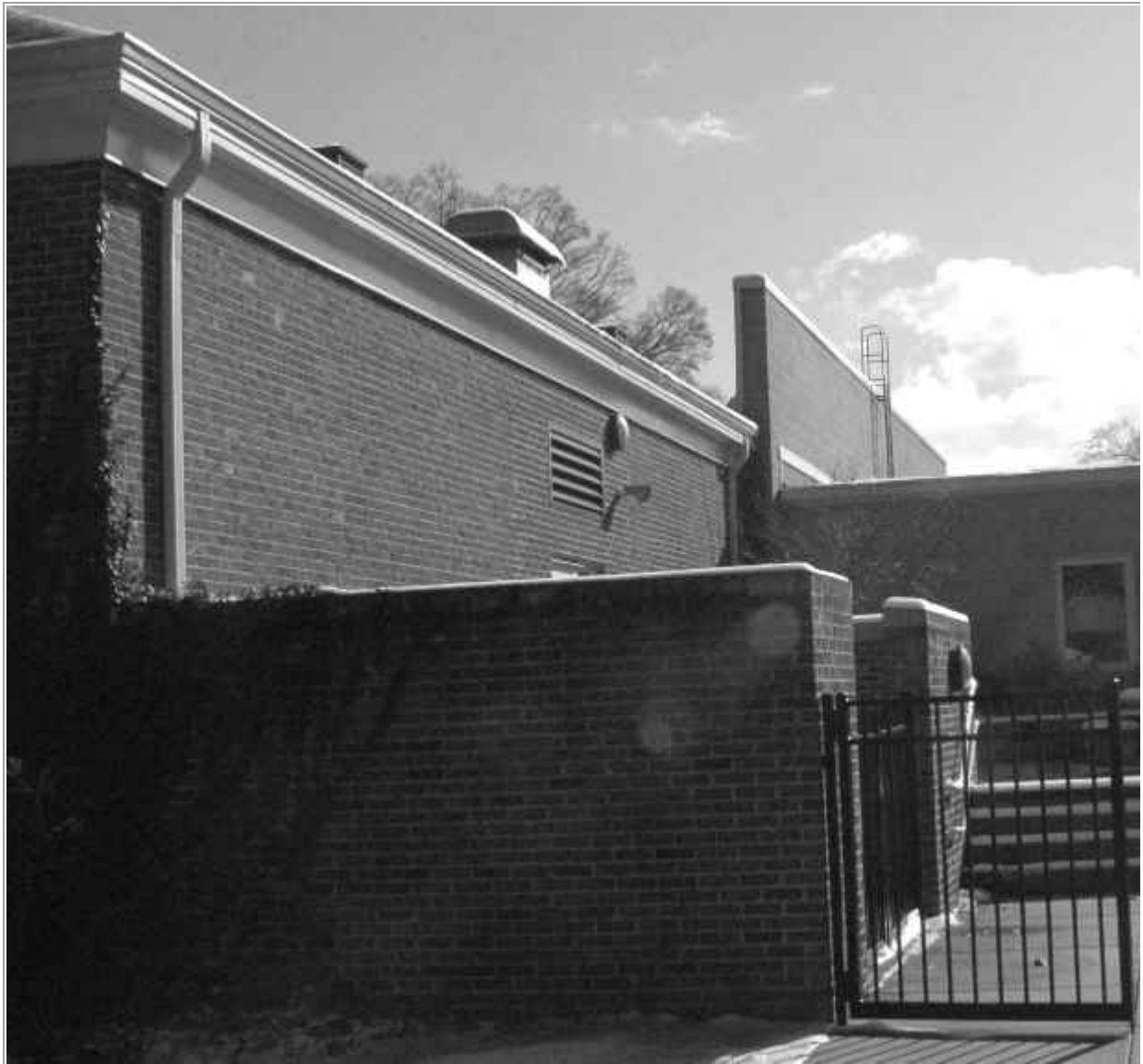
The rear of the 1935 building has been largely obscured with new construction. A portion of the original rear elevation is extant adjacent to the north elevation. A vent and new doorway may have been added. Two shed-roof dormer vent are set above the rear elevation. Various modern vents and pipes pierce the roof.
