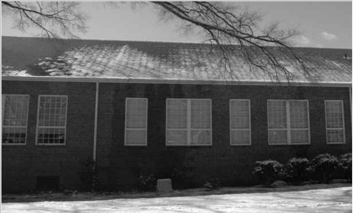
The classroom addition is very wide, spanning fourteen bays. From the north, the first seven bays contain alternating single and double twenty-over-twelve replacement windows.
