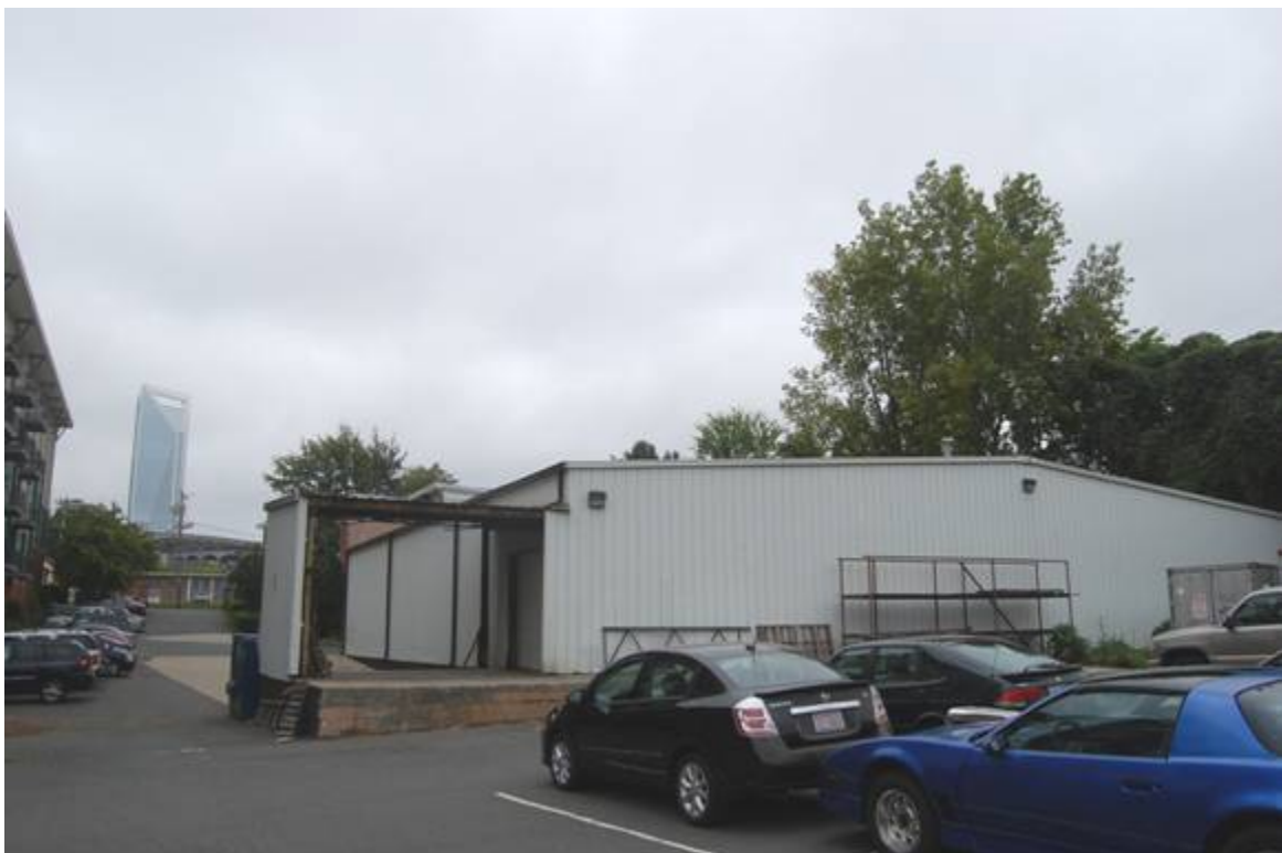
Defiance Sock Mills, Rear Warehouse, Looking East.
