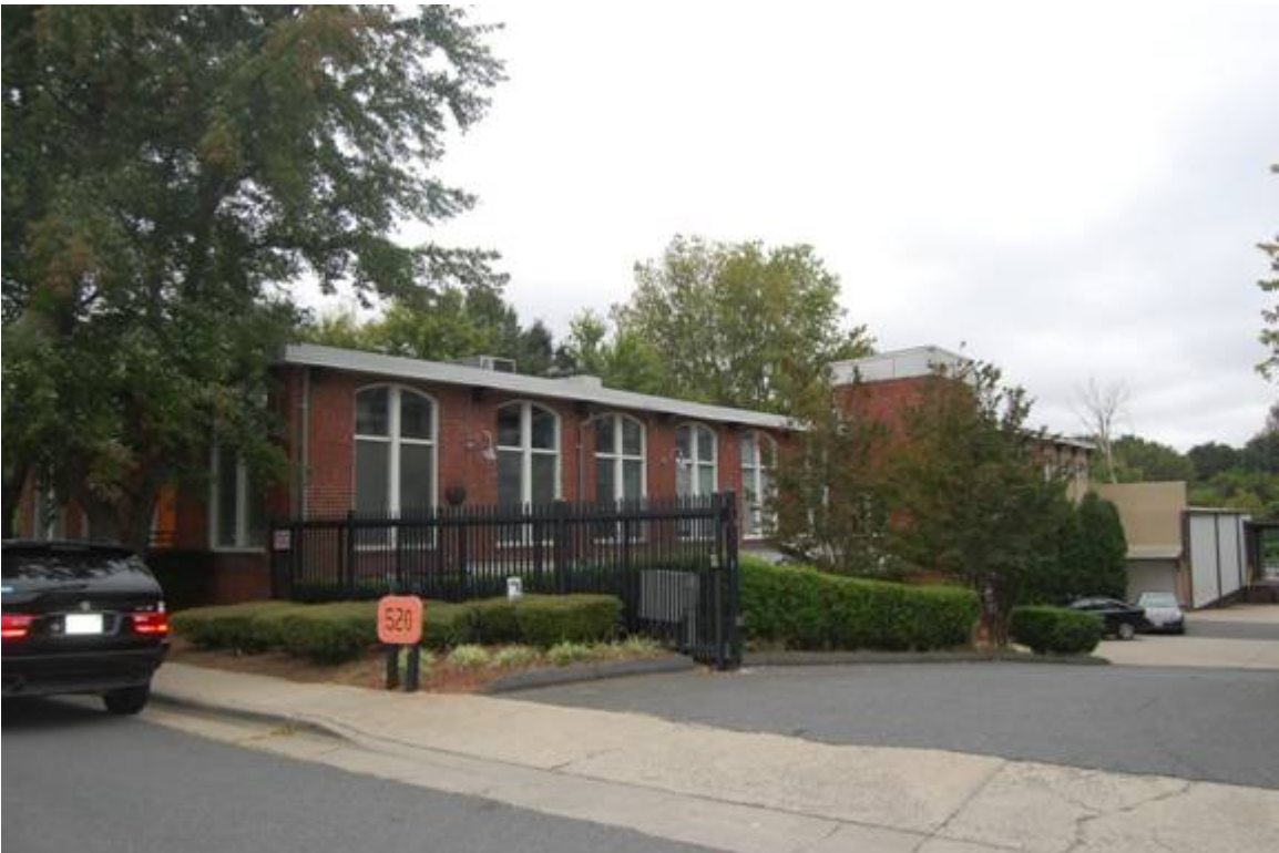
Defiance Sock Mills, Side (North) Elevation, Looking Southwest.
