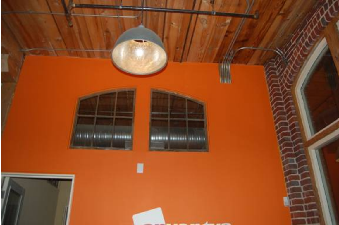
Defiance Sock Mills, Interior, Detail of Reused Original Transom Window.
