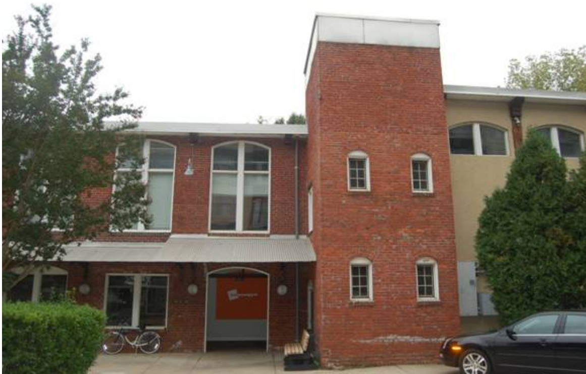
Defiance Sock Mills, Side (North) Elevation Entrance and Stair Tower, Looking South.
