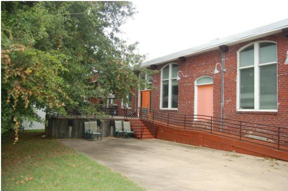
Defiance Sock Mills, South Elevation and Loading Dock, Looking Northwest.
