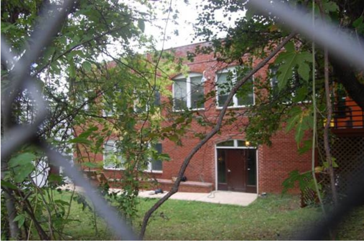
Defiance Sock Mills, South Elevation of Mid-section, Looking North from P&N Railway Line.
