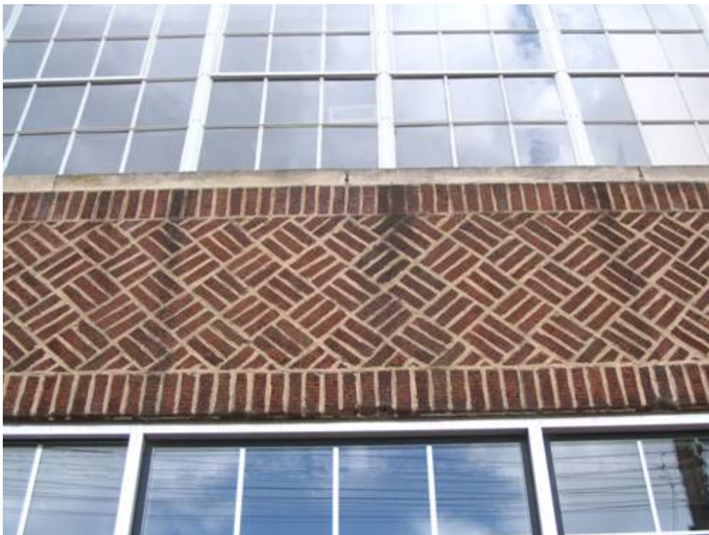
Crane Company Building, Main Elevation, Herringbone Brickwork.
