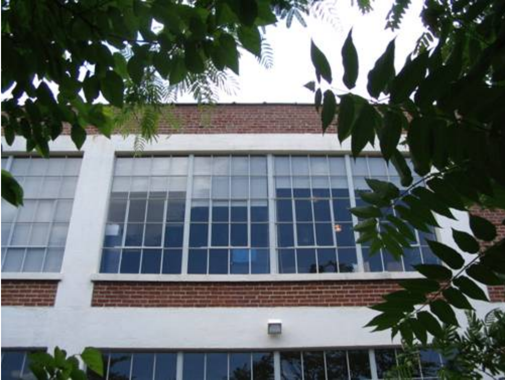
Crane Company Building, West Elevation, Windows, Looking East.
