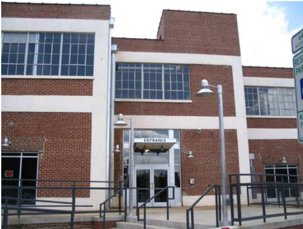
Crane Company Building, Rear (South) Elevation, Looking North.
