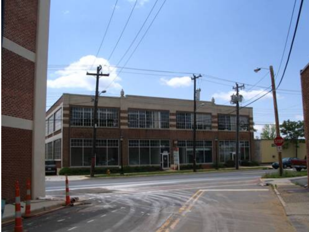
Crane Company Building, Main (north) Elevation, Looking South.
