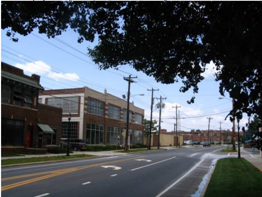
Crane Company Building, Main Elevation, Looking West along West Morehead Street.
