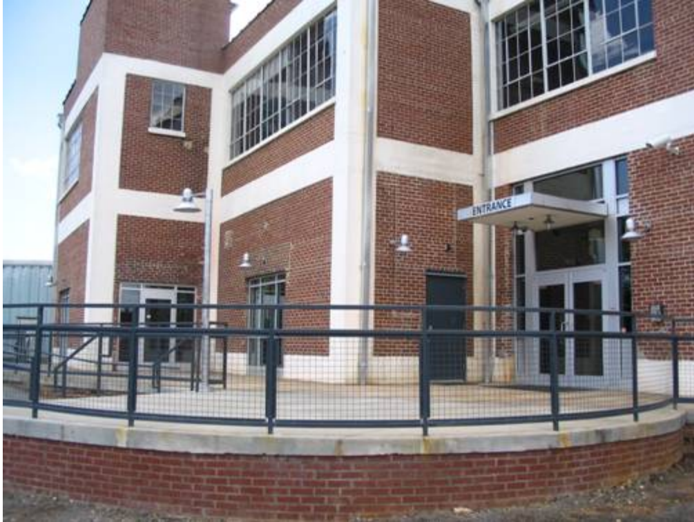
Crane Company Building, Rear (South) Elevation, Looking West.
