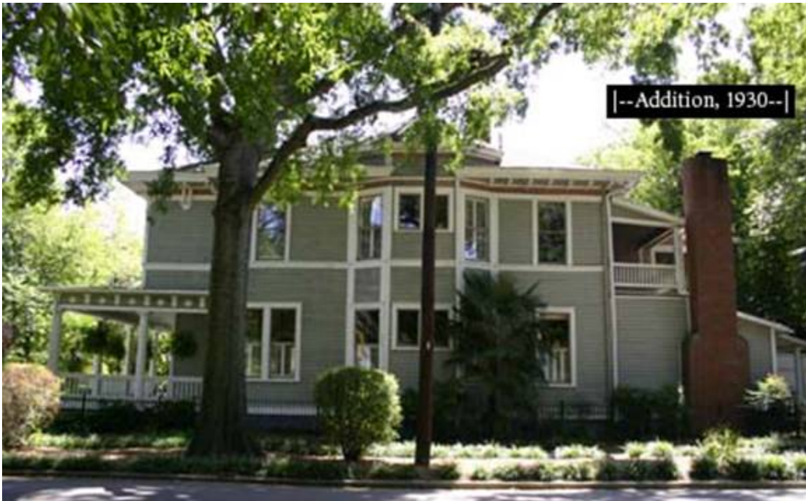
The northwest elevation
