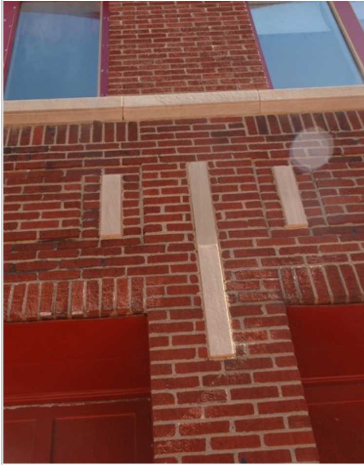
Detail of facade shows trim, brickwork and steel lintels.
