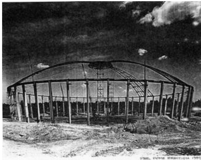
Dome under construction ca. 1954
