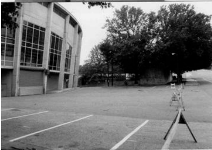
Service Area Located off Coliseum Drive on West Side of Building
