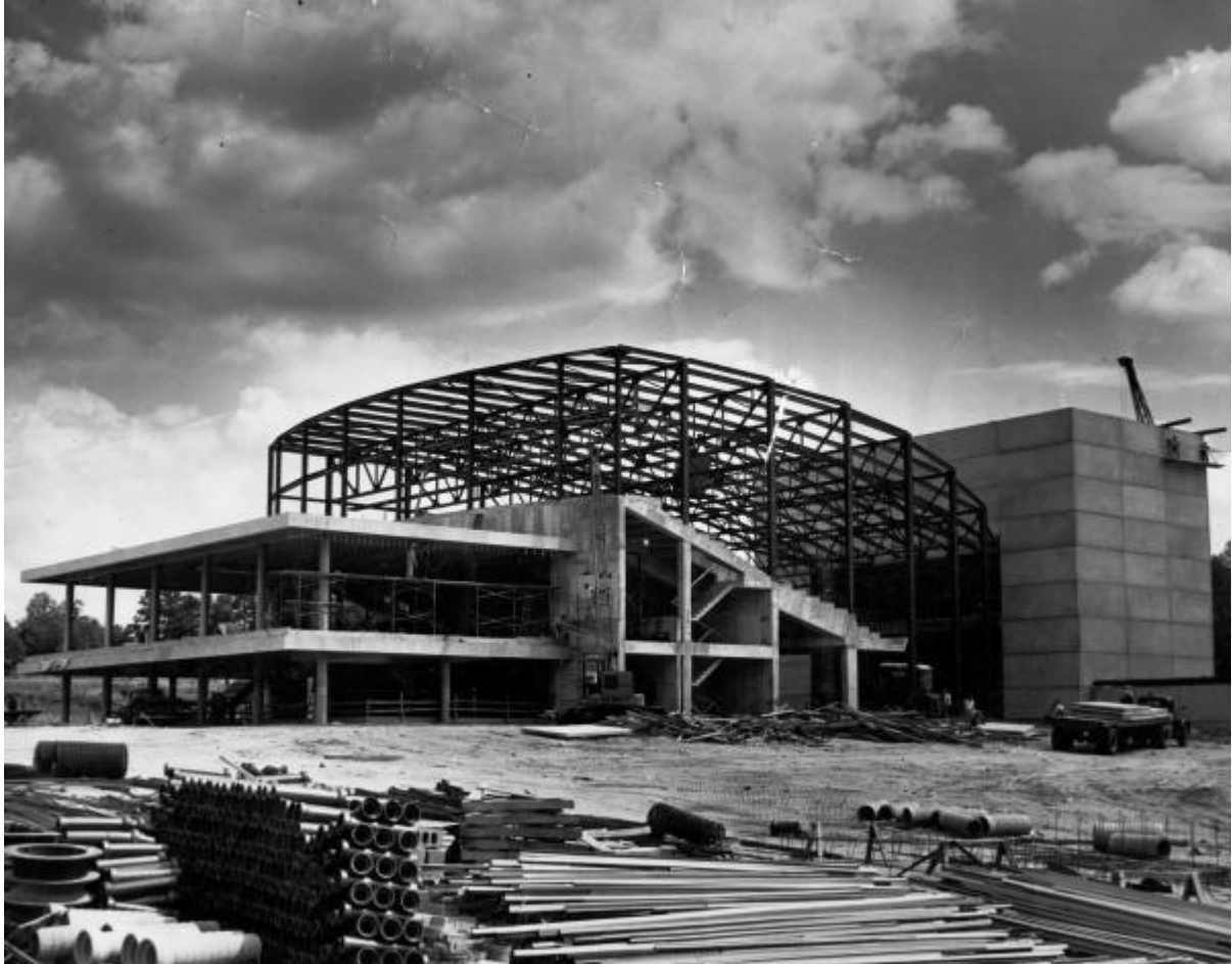
Ovens Auditorium under construction, photograph taken on July 22, 1954
