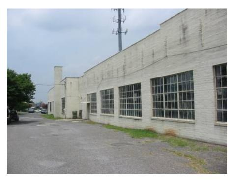
The utilitarian side and rear elevations have concrete brick walls, capped at the roof line by terra cotta coping, and punctuated by banks of steel sash factory windows and pedestrian doors. The rear elevation has a central loading bay with a modern overhead door and a boarded over window. The northwest corner of the rear elevation is contiguous with the added rear wing. The concrete block addition has a gable roof and several loading bays.
