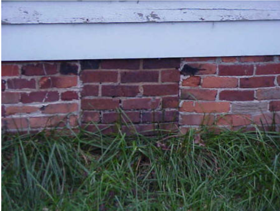
Original brick pier with in-fill curtain foundation walls
