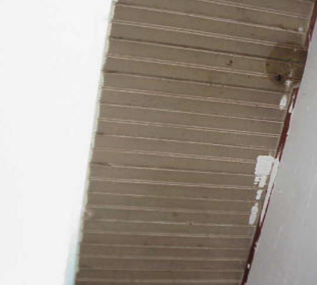
A beaded-board ceiling is intact above a later ceiling
