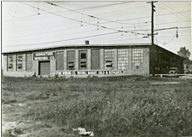
Armature Winding Company Building from across Piedmont and Northern Railroad tracks.
