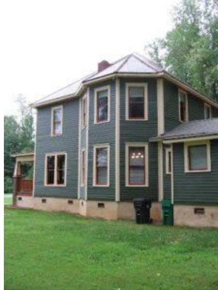
The north elevation of the Abernethy house is two bays wide. The left bay has paired windows on the lower story and a single window on the upper story. These windows are centered within the bay. A low brick chimney is set approximately centered between the two bays. The right bay features a three-sided two story projecting bay topped with a slate hip roof. Reminiscent of the Queen Anne Style, this element has single windows on both the lower and upper stories centered in each side of the bay.
