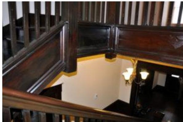
The staircase leading up the second story is fully original. Bullnosed wood treads with underlying cove moulding top the risers. Moulded wood railings are supported by square balusters. Square newel posts, which receive the railings, feature wood trim just below the railings and moulded caps. The posts extend past the the ceiling of the first story. The staircase framing as well as the stringers are accented with wood panels and curved moulding.
