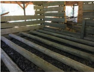
These photos show the current condition of "Cabin A" - The four walls are free standing and the floor joists have been placed. A hearth has been cut from one wall, a functioning fireplace will be constructed when the cabin is moved to its final location.
