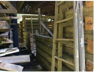
These photos show the current condition of "Cabin B" - As with it's neighbor, the four walls are free standing and the floor joists have been placed. A hearth has been cut from one wall, a functioning fireplace will be constructed when the cabin is moved to its final location.
