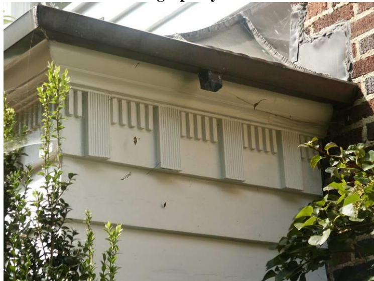
Figure 10 - Dentil molding – used on the front façade, rear elevation and side porch cornices. Photograph by Diane Althouse.
