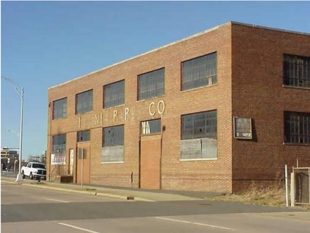
The five-bay wide south elevation is relatively symmetrical. The three large first-story window openings are filled with 72-light metal-frame windows. Between the windows, two large door openings topped with 16-light transoms, have been infilled with brick. The five second-story windows are the same triple 16-light windows found on the facade. A single doorway with a brick stoop and steps has been cut into wall between the westernmost window and original industrial door.
