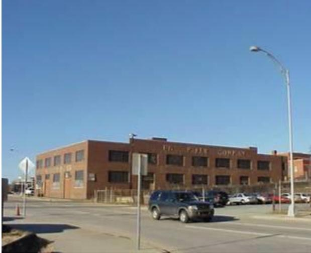
The Virginia Paper Building employed fire-proof construction. The solid brick exterior walls surround reinforced concrete slab floors and roof, which are supported by poured concrete mushroom columns. These noncombustible materials combined with metal frame doors and windows, resulted in a virtually fire-proof building shell. These elements of a fire-proof design became popular in the 1920's and were the culmination of over one hundred years of technical advances.
