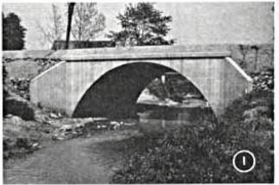
Bridge across creek.
