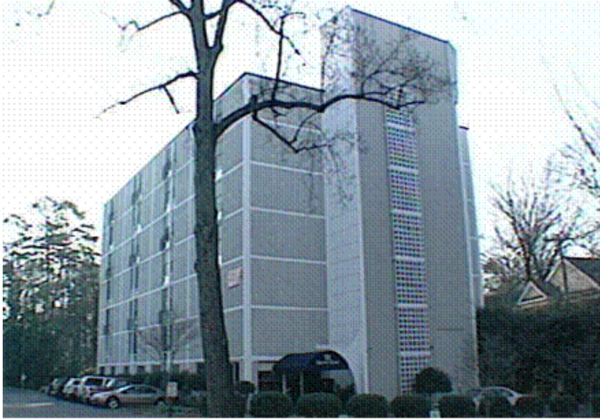
Sutton House at 511 Queens Road
