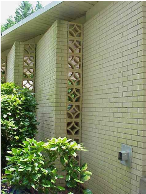
Detail of the carport
