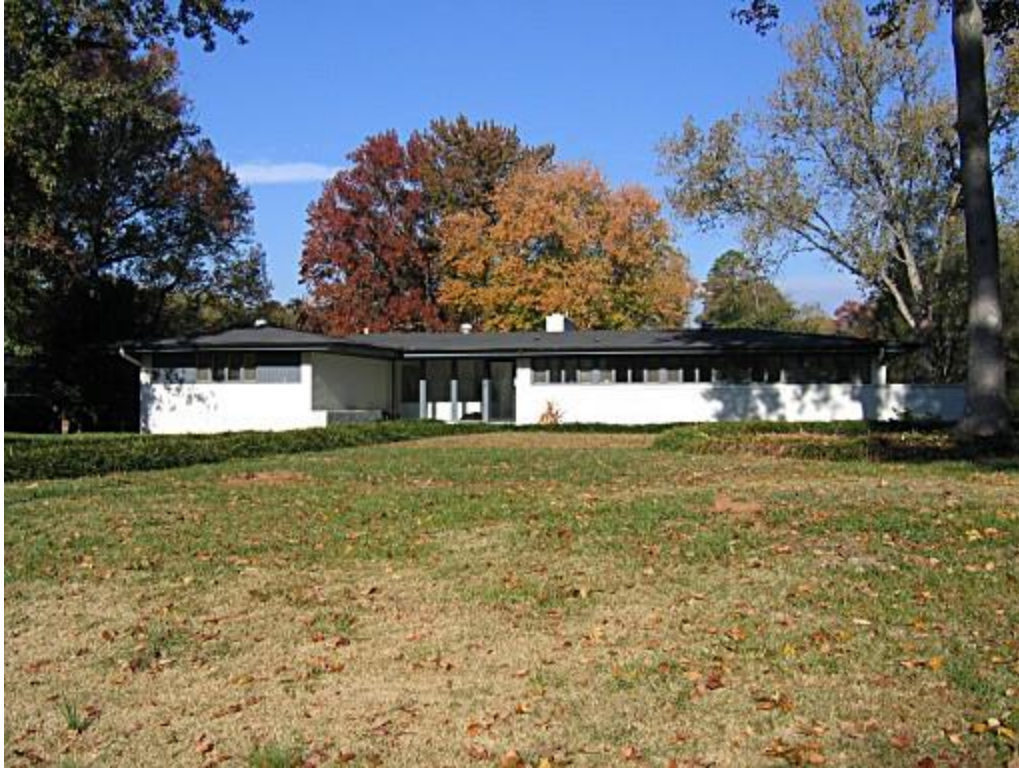
This home on Cloister Drive illustrates the nature of home sites.
