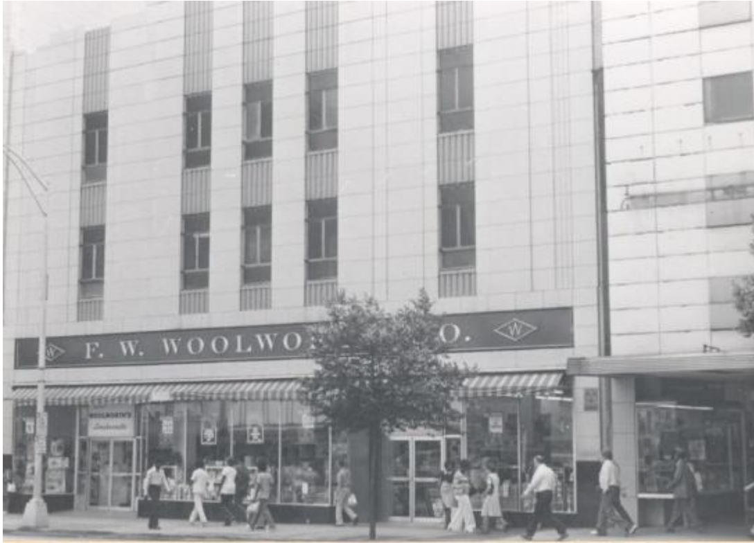
Charlotte has lost many of its older center city eateries, including the lunch counter in the F. W. Woolworth Store on N. Tryon St. (above) and the S. & W. Cafeteria on W. Trade St. (below). Both demolished.
