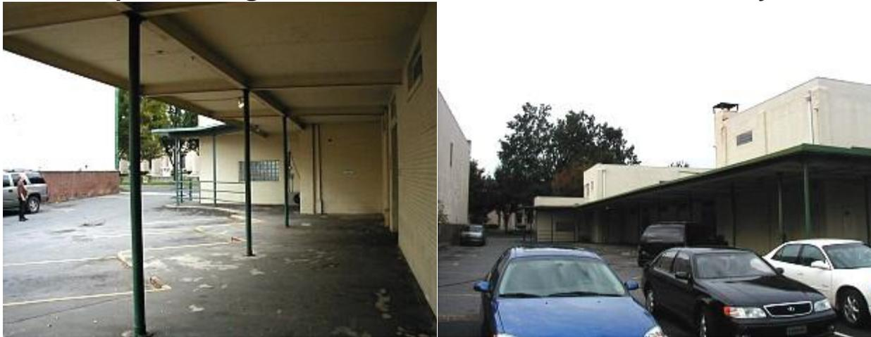
The east, west, and south elevations are completely unadorned except for the metal canopies running along the length of all three elevations. The canopies are supported by thin, round metal columns that are regularly spaced underneath the canopies. A parking lot lies along the east and north elevations of the building.
