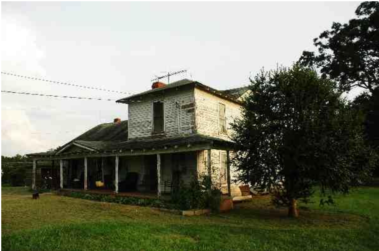
This August 2005 photograph shows the major modification to the Bell House that was made about 1913. A large, gable-roofed rear addition was completed and became essentially the new front of the house. The original front porch was removed, and a new porch was built on the new front.
