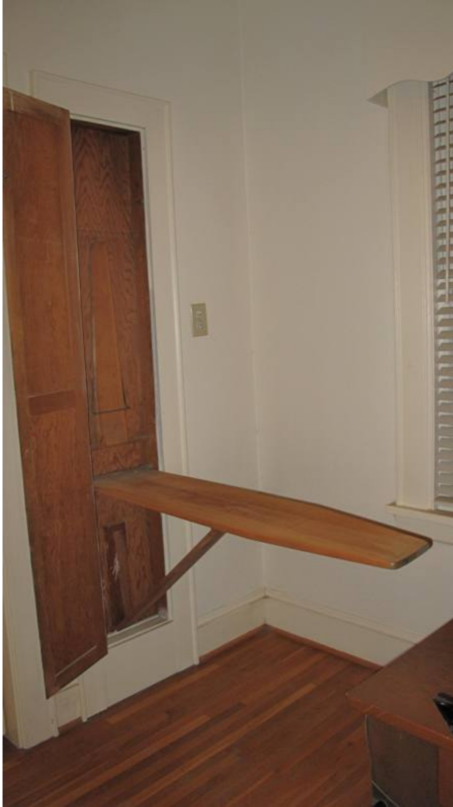
The integrity of the interior of the Stratton House is enhanced by the presence of many other features that are typically removed or replaced in early-
