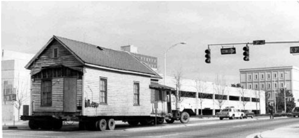
Shotgun house en route to its new location
