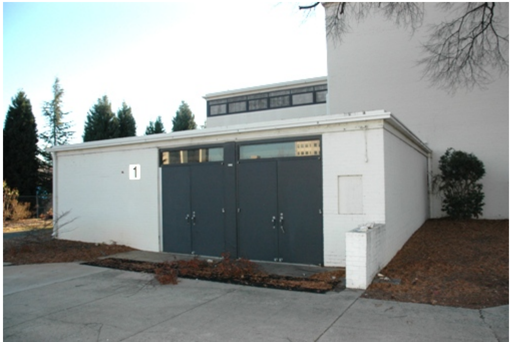
Gymnasium vestibule/box-office. The metal doors are located in an area that was once an open recessed porch. The narrow box-office to the right of the doors is original.
