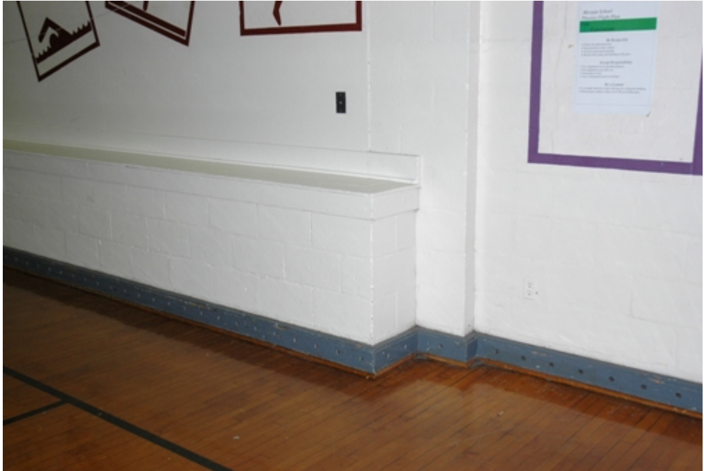
Detail of projecting stage floor. The original hardwood gymnasium floor features an unusual ventilated baseboard that allows the large expanse of wooden floor to expand and breathe.
