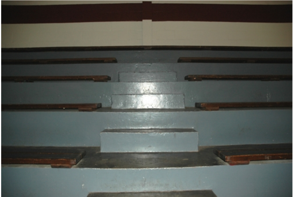
The concrete bleachers and steps were formed in place.
