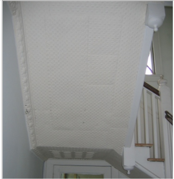
Metal covering stair soffit
