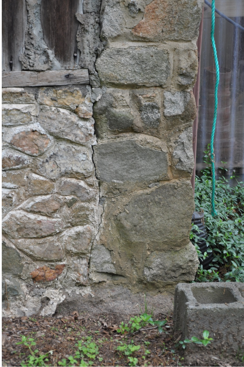
Figure SEQ Figure \* ARABIC 2 – Individual stone piers are visible within the foundation wall.
