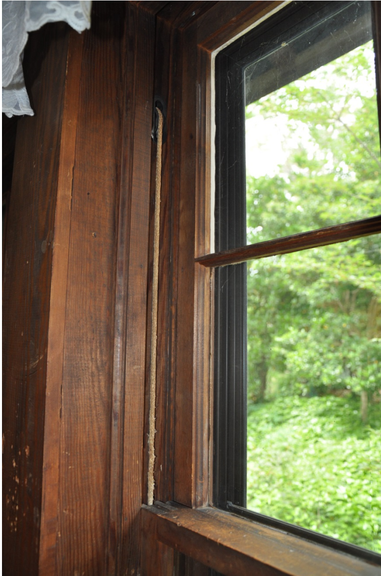
Figure SEQ Figure \* ARABIC 4 - Typical original double-hung wood sash window, exterior and interior views. Storm windows have been installed on the exterior.
