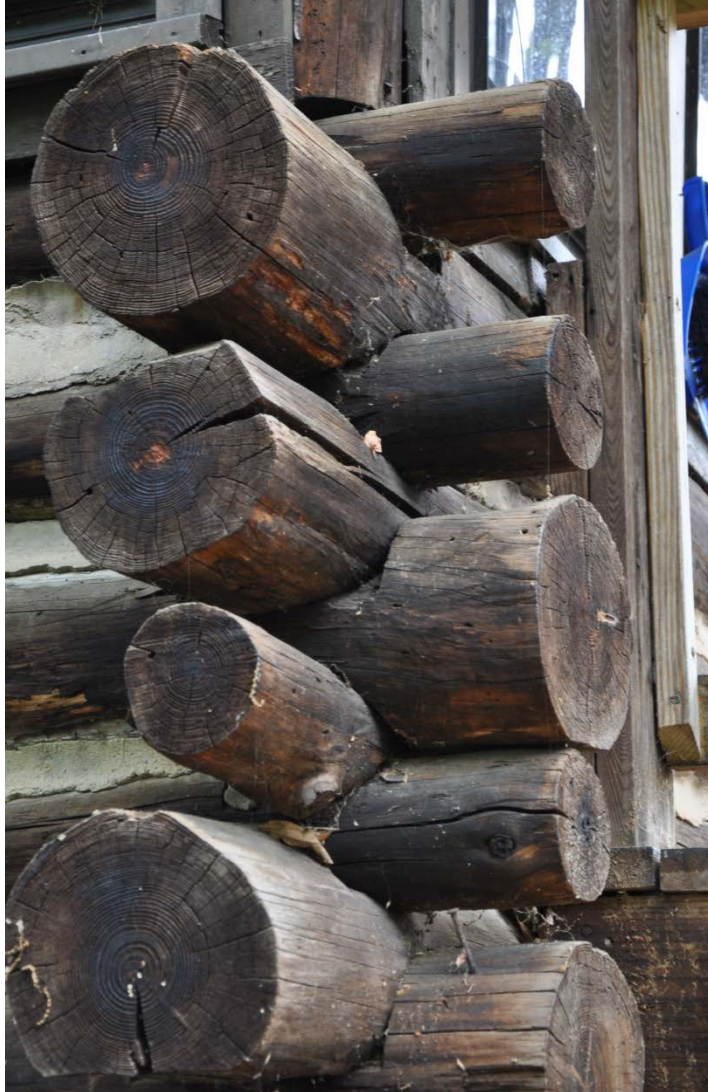
Figure SEQ Figure \* ARABIC 3 - This typical corner detail shows the extended logs sitting in saddle notches.
