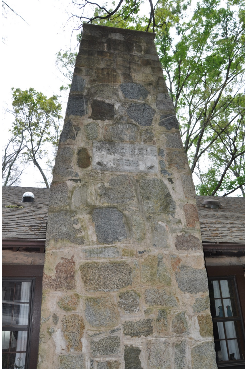
Figure SEQ Figure \* ARABIC 7 - Stone rubble chimney on the north elevation.
