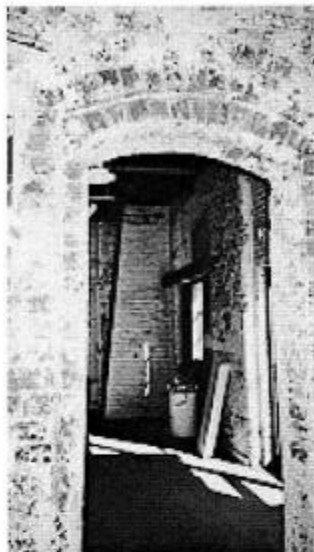
Interior door illustrates chamfered bricks
