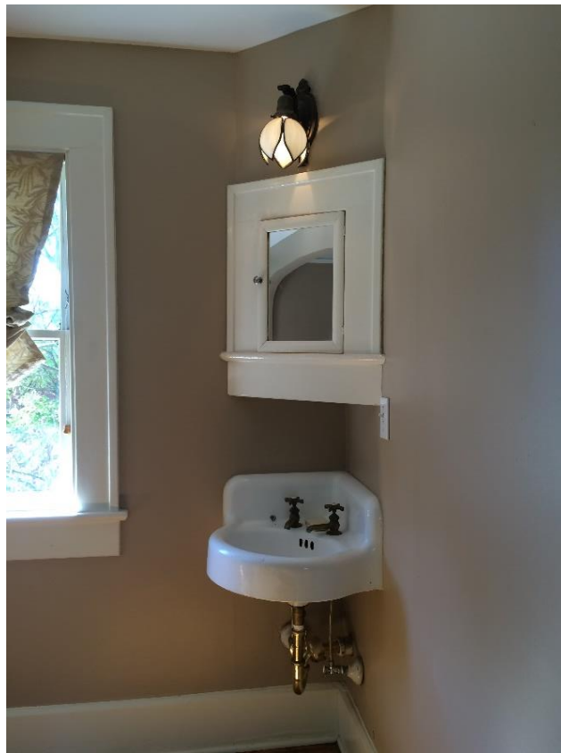
Upstairs Corner Sink
