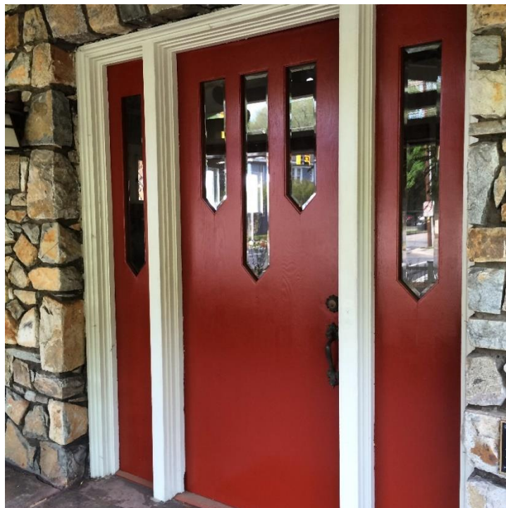
Original Front Door
