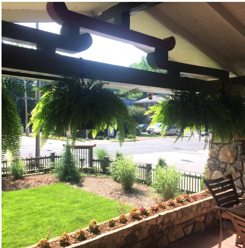
Front Porch Rafters
