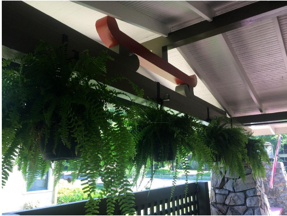
Side Porch Rafters
