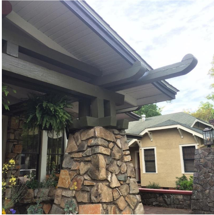
Japanese-Inspired Curved Rafters on Front Porch
