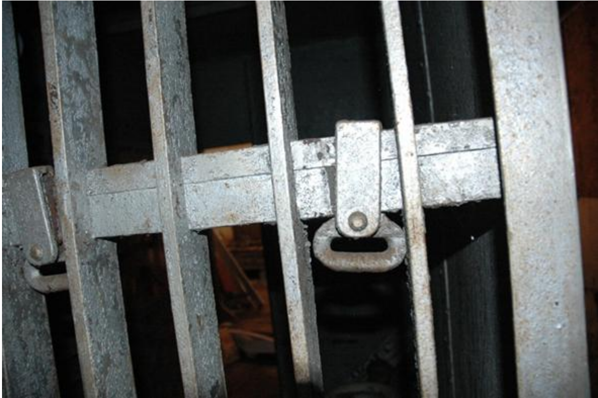
Detail of restraint bracket.
