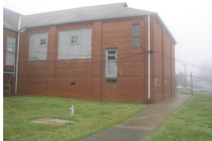
Rear wing houses the auditorium.
