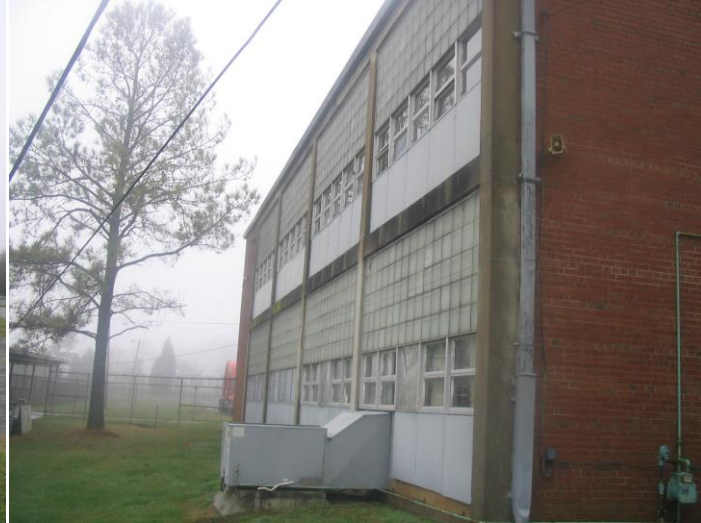
East (rear) Elevation of South Wing
