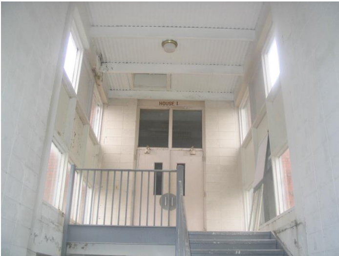
Masonry Hyphens Attach Old and New Sections
