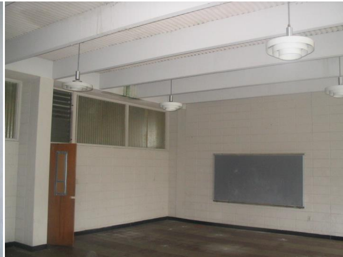
Second Story Classroom in South Wing
