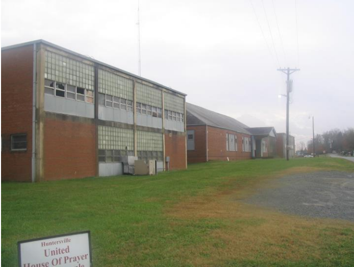
West Elevation of North Wing
