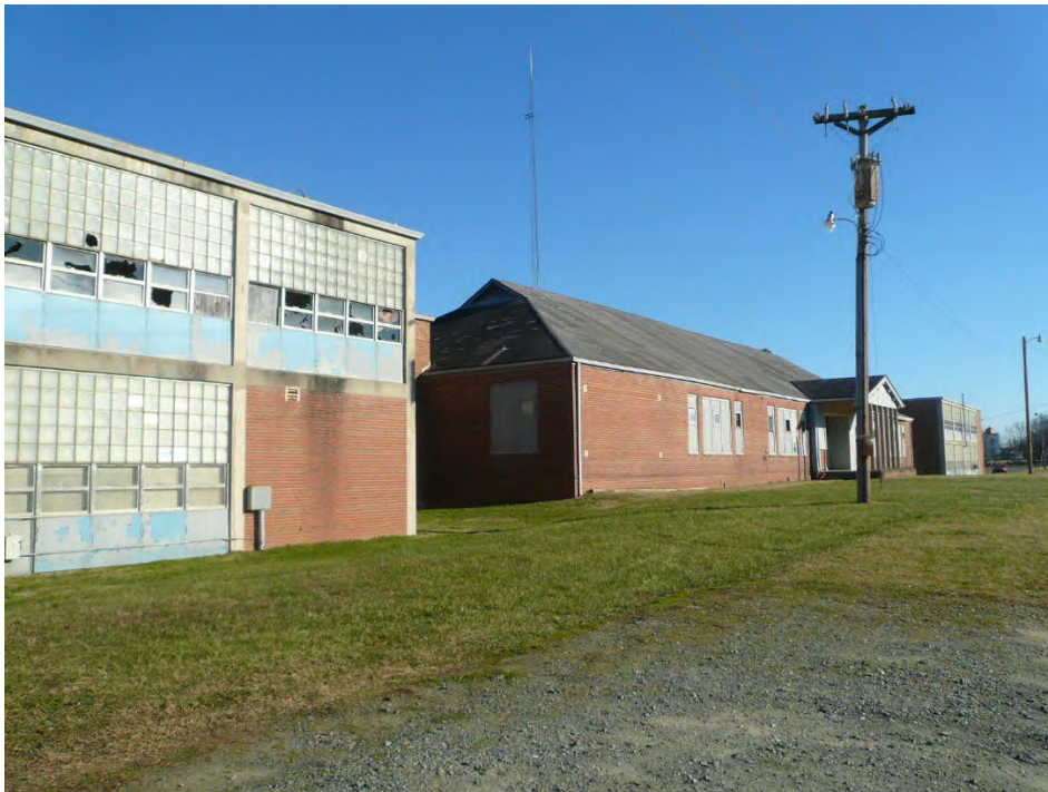
Figure 1: Historic 1937 building in center
